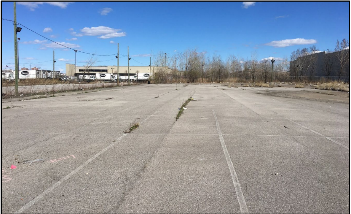
Photo 7. Facing east in the western portion of the Fish Market parking lot. The engineering cap remains in place with some vegetation growing through cracks in the asphalt.
