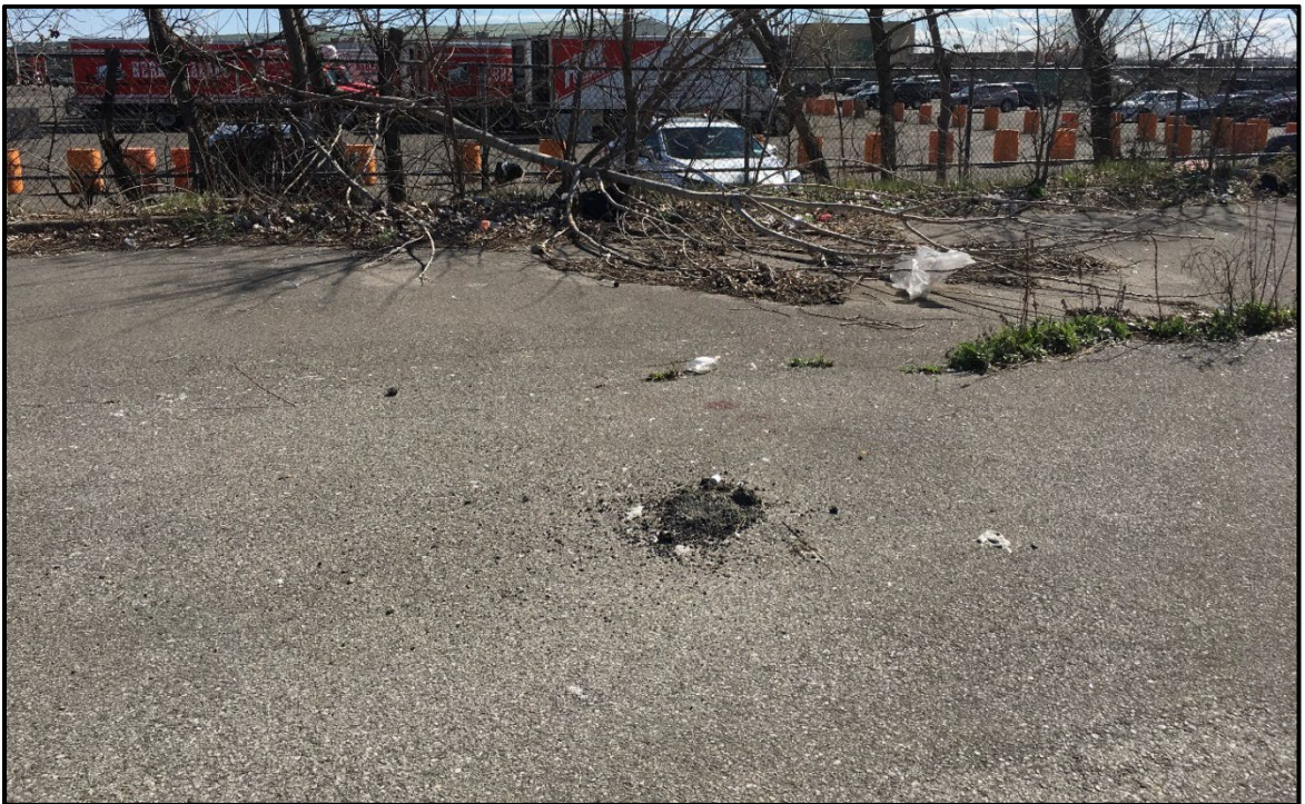
Photo 6. Facing south; the southeastern corner of the Fulton Fish Market parking lot. A former geotechnical boring backfilled and patched at grade.
