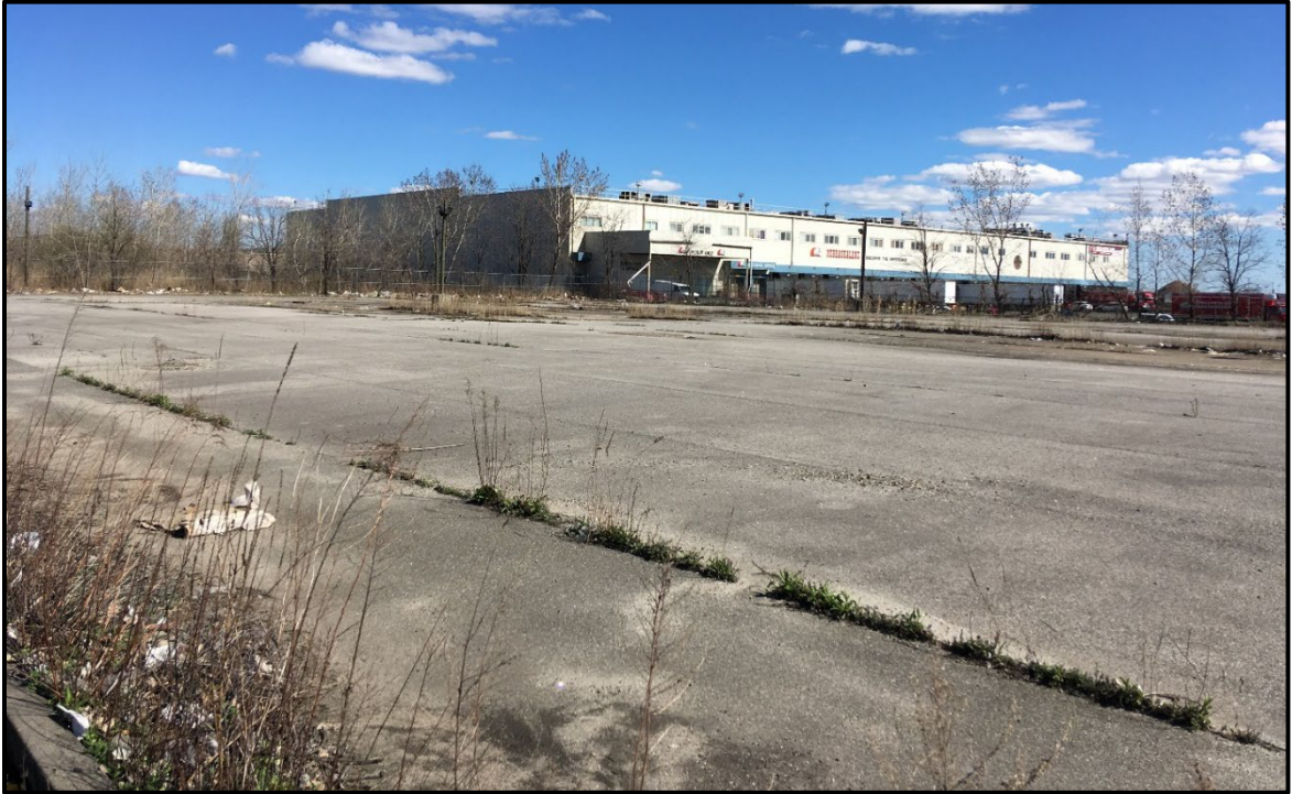
Photo 5. Facing southeast; the paved parking lot in the northern portion of Site A OU-1. The engineering cap remains in place with some vegetation growing through cracks in the asphalt.
