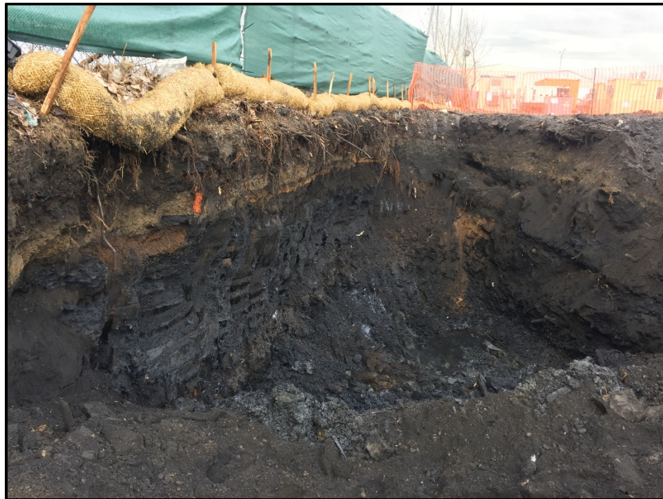
Photo 8. Facing south along the western boundary of Site A OU-1 during the BCP Site A-2 remediation (January 2018). Deposit of coal tar impacted fill material in the sidewall adjacent to the unused walkway between Site A-2 and the Meat Market/Nebraskaland parking lot.
