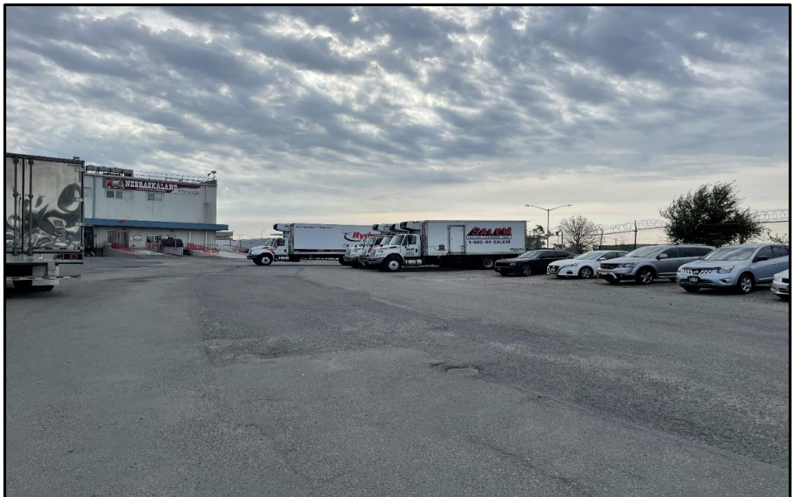
Photo 4. Facing southeast in the Nebraskaland paved parking lot.; evidence of general wear from vehicular traffic. Minor cracking and potholes present.
