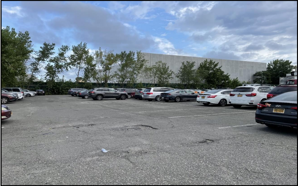
Photo 7. Facing northwest in the western portion of the Nebraskaland parking lot. Minor potholes and cracking present.
