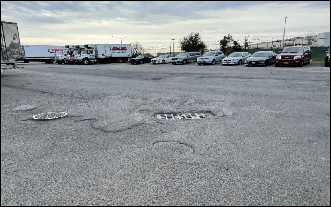
Photo 3. Facing southeast within the paved parking lot adjacent to Nebraskaland. Asphalt in fair condition and evidence of former patching.
