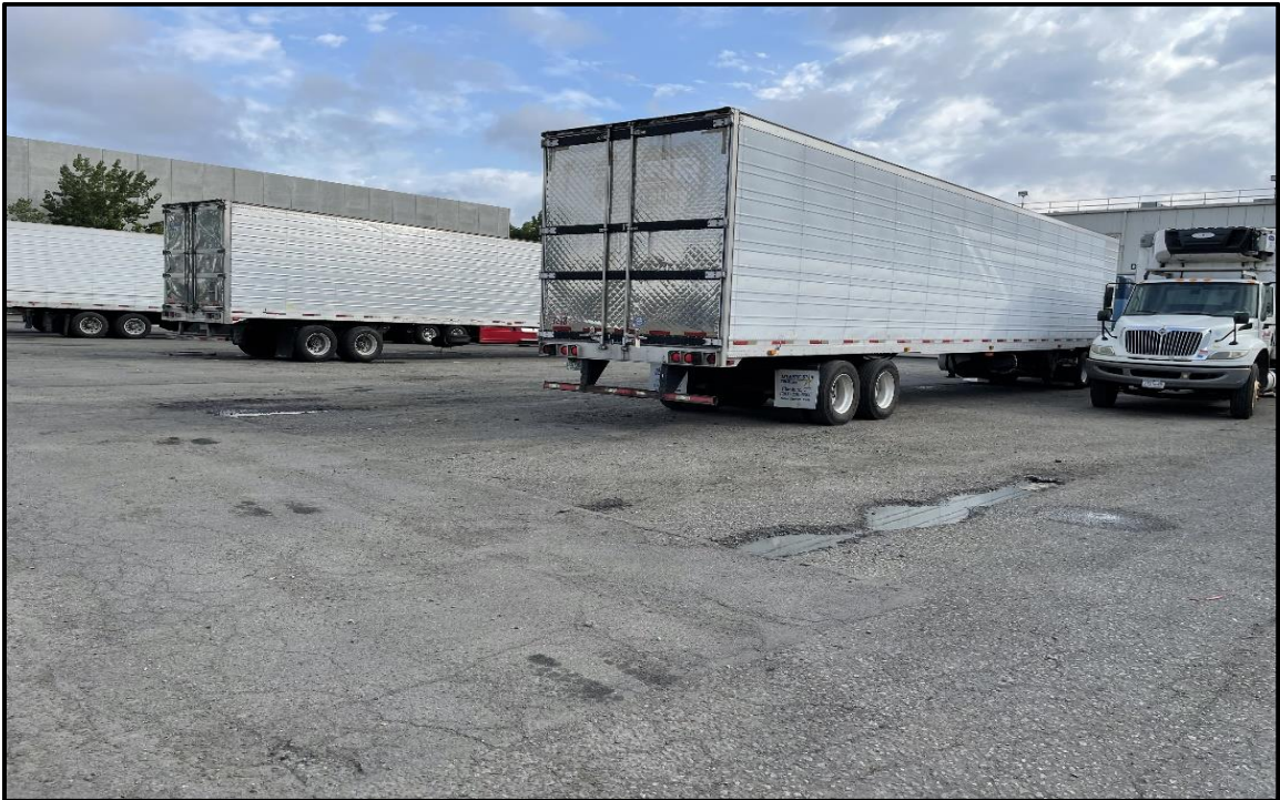
Photo 8. Facing northeast within the paved Nebraskaland parking lot; shallow potholes with some standing water noted.
