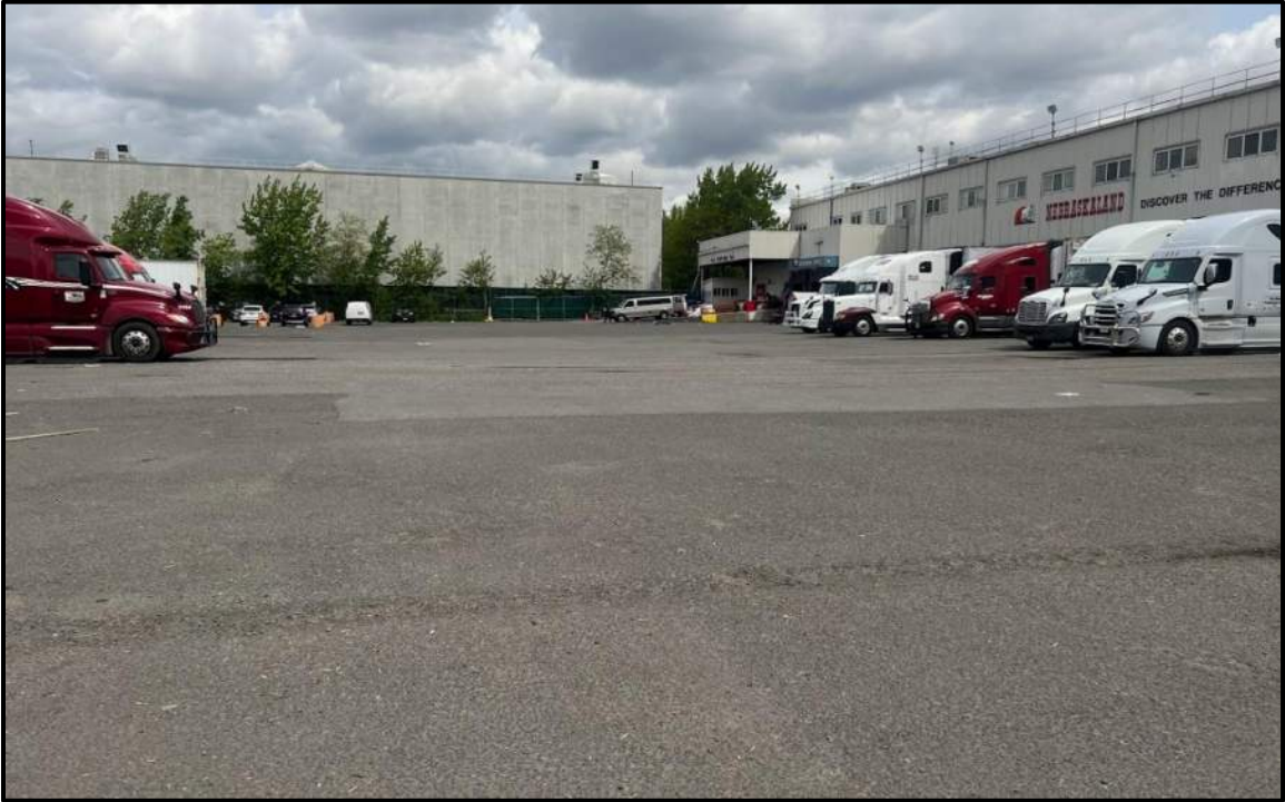
Photo 3. Facing north within the paved parking lot adjacent to Nebraskaland. Asphalt in fair condition and evidence of former patching.
