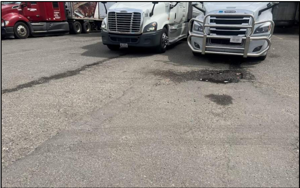
Photo 6. Facing east; loading dock in the eastern portion of the Nebraskaland parking lot. Minor cracking and potholes noted.
