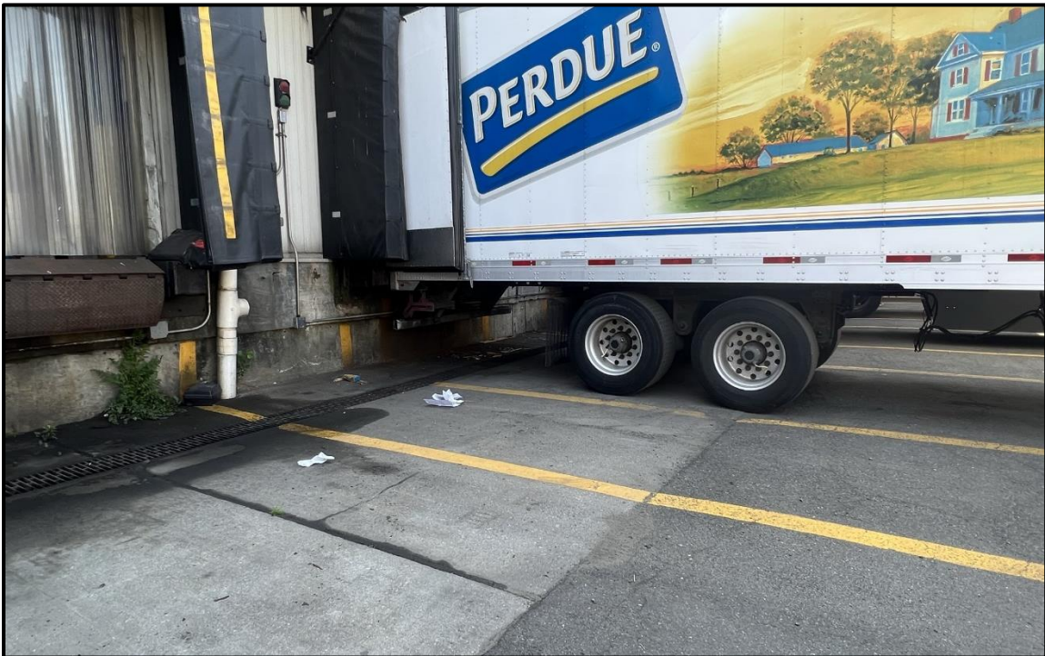
Photo 6. Facing southeast along the Nebraskaland loading dock; reinforced concrete slab in fair condition with minor asphalt cracking noted.
