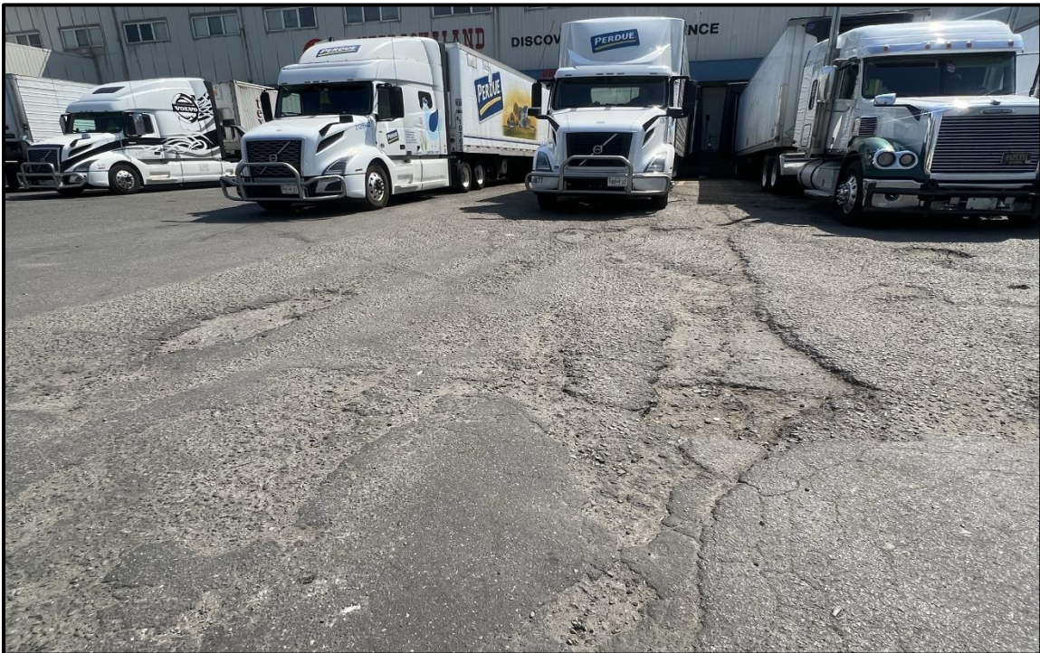
Photo 4. Facing east in front of the Nebraskaland loading dock; larger cracks and potholes noted, former patched area (left) in fair condition.
