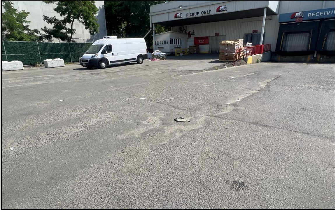
Photo 7. Facing east towards the Nebraskaland Pickup loading dock; minor cracks and potholes noted from vehicle traffic.
