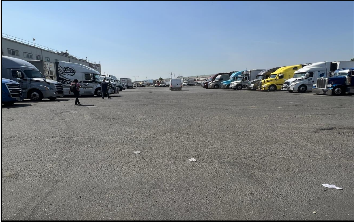
Photo 3. Facing south within the truck loading area of the paved parking lot, adjacent to Nebraskaland. Asphalt in fair condition, with minor cracking and potholes present.
