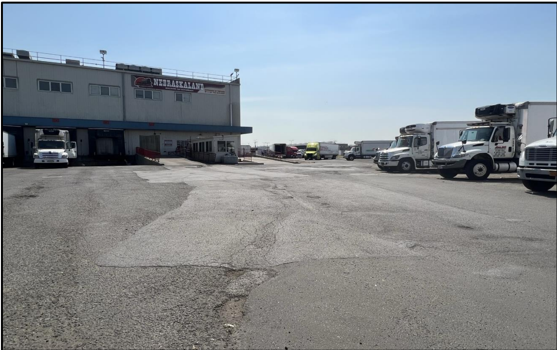
Photo 2. Facing southeast adjacent to Nebraskaland; the southern portion of the paved parking lot and internal roadway within the Meat Market facility showing minor wear and potholes from vehicle traffic, as well as former asphalt patching.
