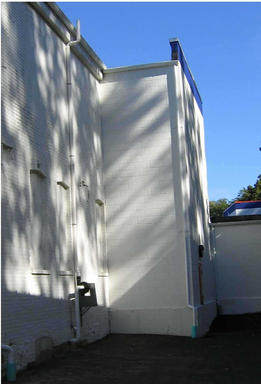
Exhaust Fan 5, Building 7
