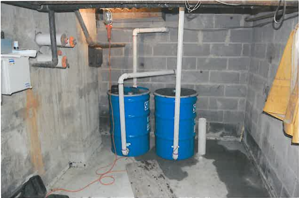
TWO LIQUID-PHASE CARBON FILTERS IN SERIES
