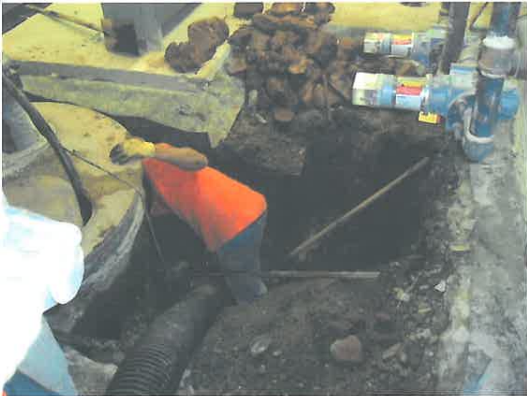
EXCAVATING SOIL IN EQUIPMENT ROOM
