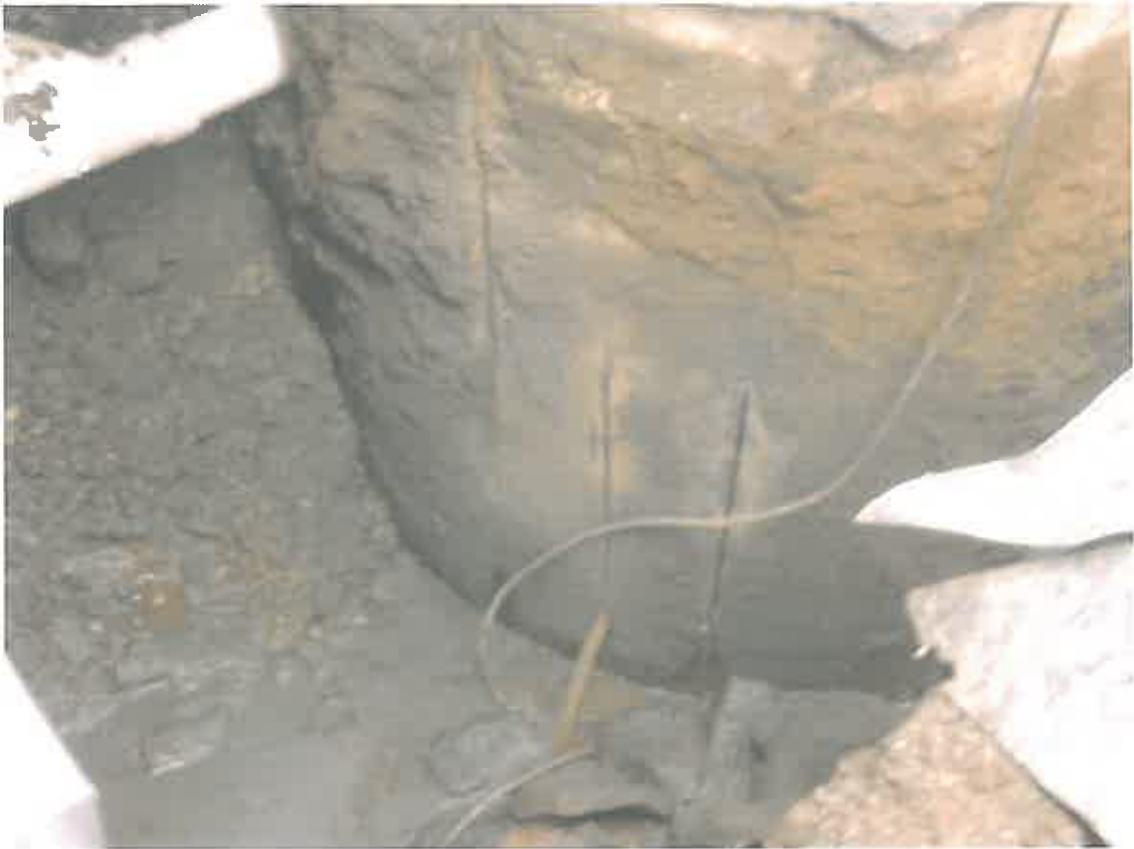
SLOTS CUT IN SIDE OF LARGE SUMP PIT
