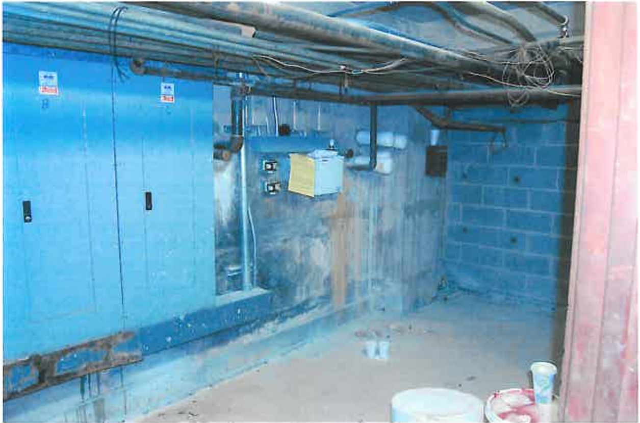
WEST ROOM, PRIOR TO 2009 IRM
