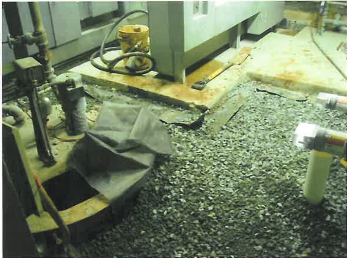
EQUIPMENT ROOM BACKFILLED, NOTE VERTICAL PIPE
