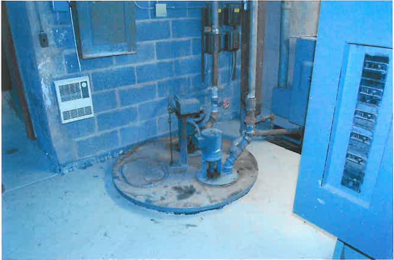
LARGE NORTH SUMP PIT IN EQUIPMENT ROOM, PRIOR TO 2009 IRM
