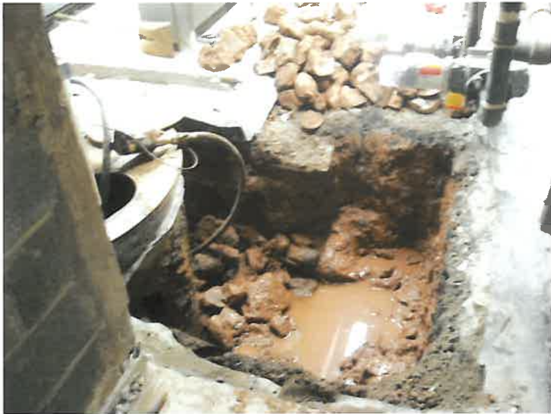
CONTINUED EXCAVATION, NOTE COBBLES
