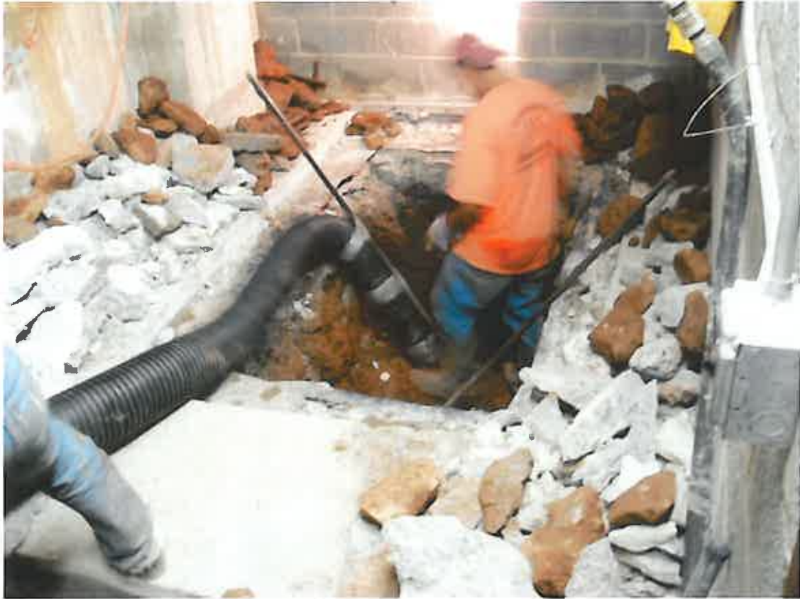
EXCAVATING WEST ROOM
