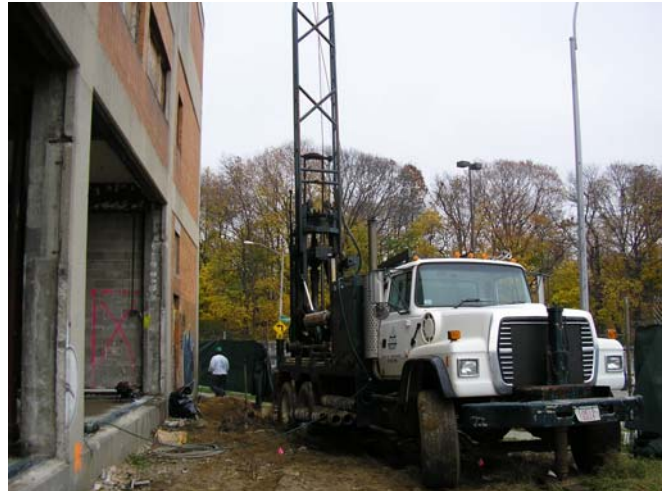
Photo #2 – View of remedial system well installation.
