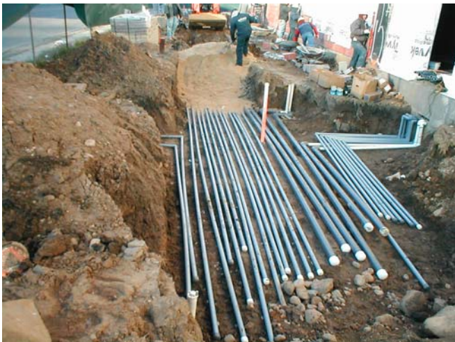
Photo #3 – View of remedial piping installation.
