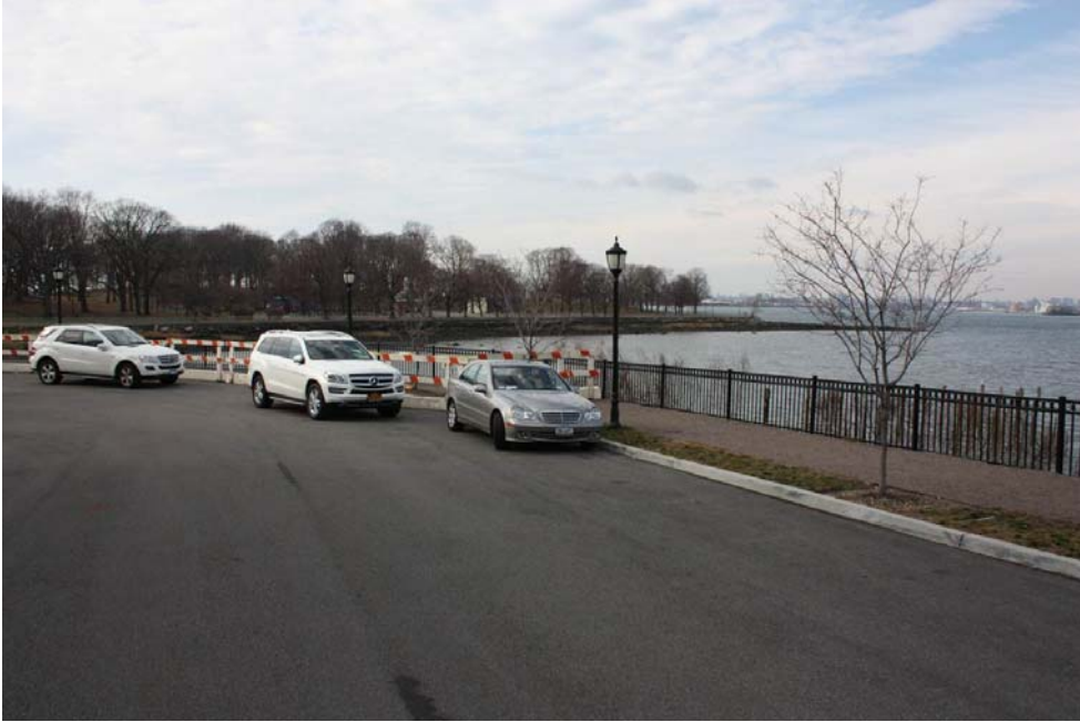
Photograph 1 – Walkway and fence sections lost to erosion of the seawall.
