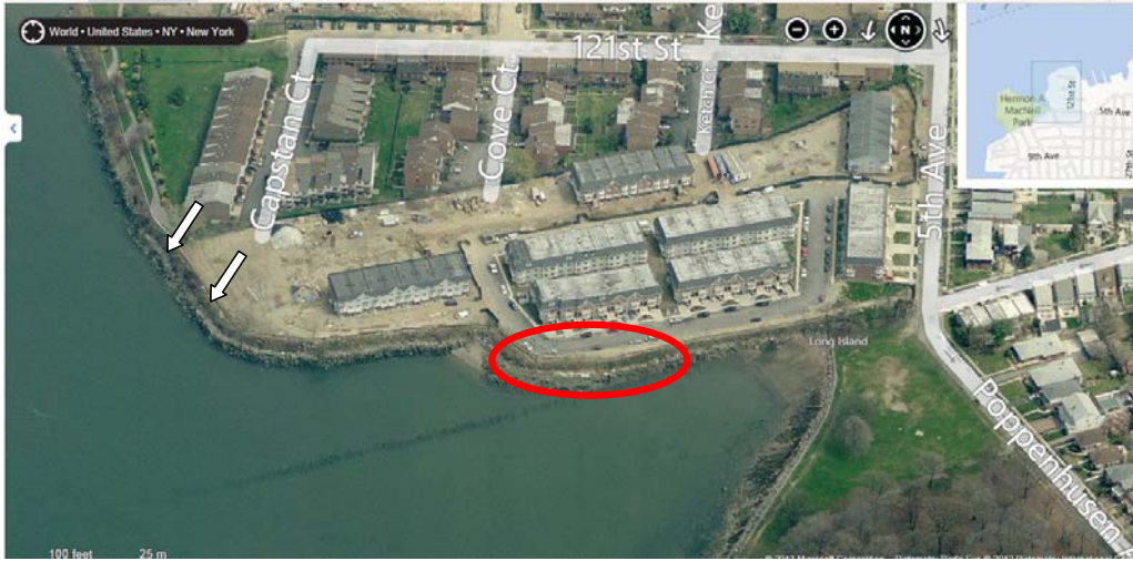
Figure 1 - Bing Maps aerial showing locations of erosion (arrows) and slope failure (red circle).
