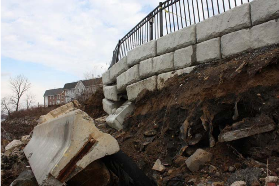
Photograph 5 – Visible strata of fill and debris evident.
