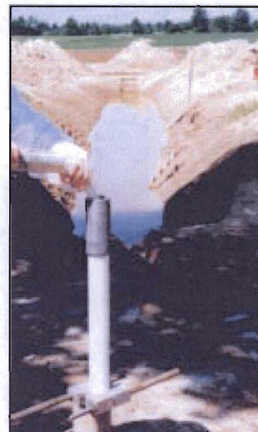
Underground oil pipeline leak assessment. Three 150 ft. (45m) installations, monitored with portable Water Level Meter and Triple Tube Sampler. Two point rising head permeability tests were conducted in each interval of the Multilevel System.
