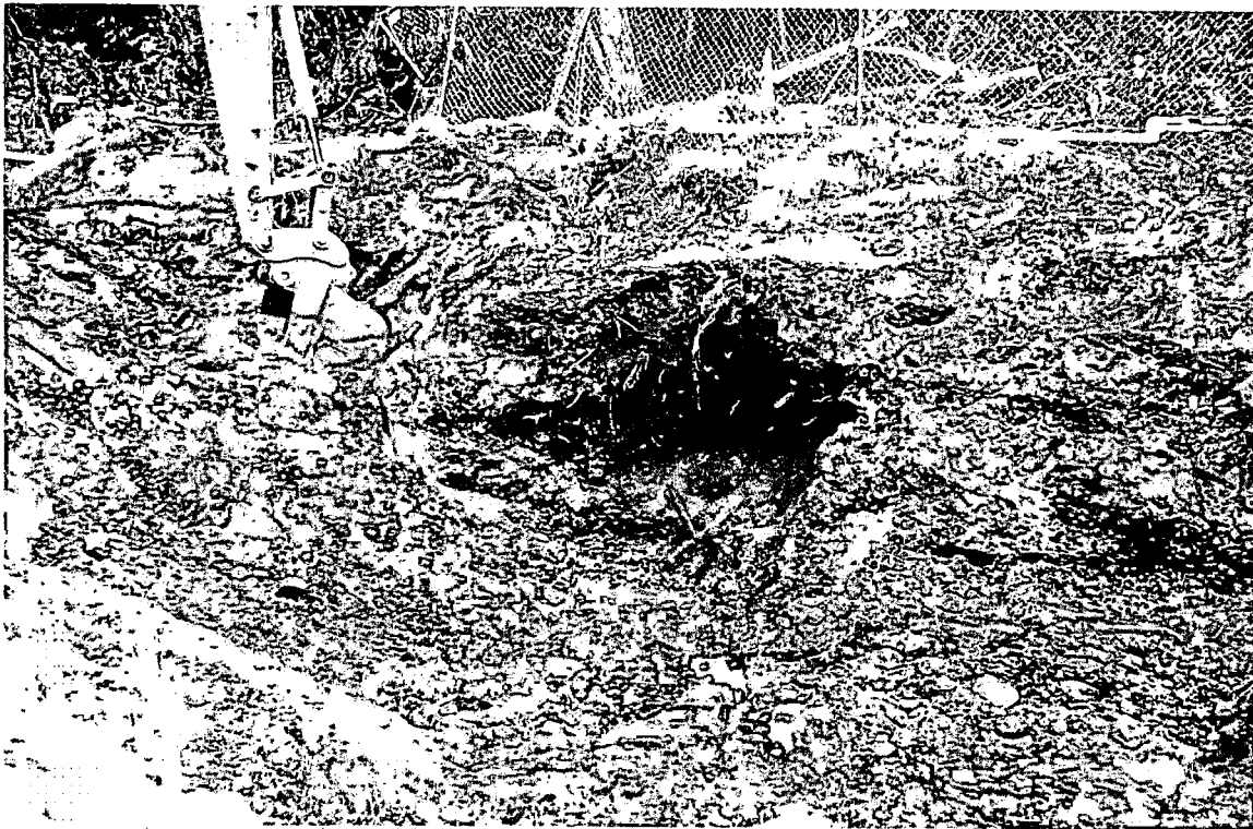
View of True Blue completing excavation in the northeast corner of the northeastern cell. The bedrock surface is the dark grey surface in the lower right corner.
