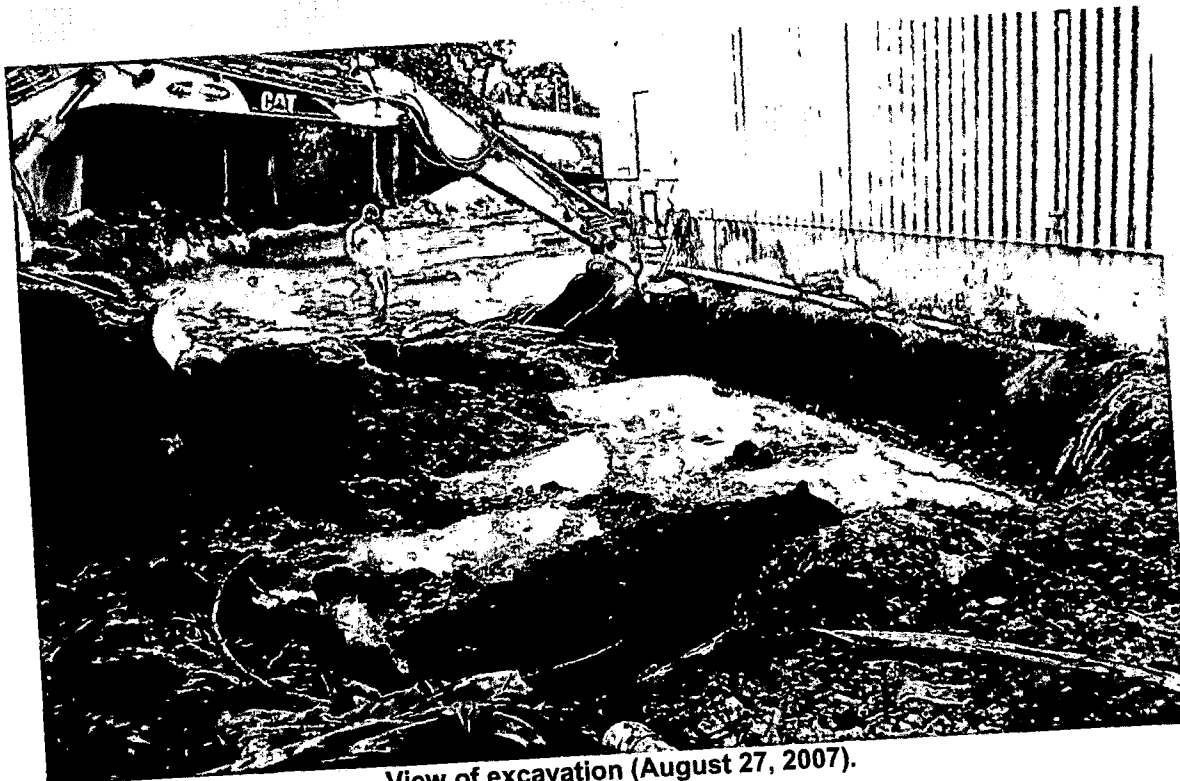
View of the excavation area after water line leak on August 24, 2007. (Water line can be seen under water in the upper left hand corner.)
