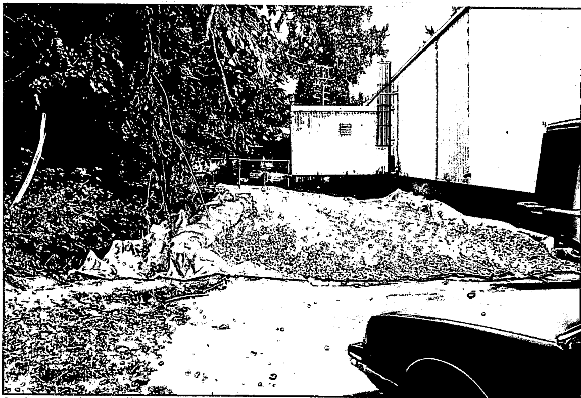
Anti-tracking pad located along the eastern side of the Dorel building, leading from the excavation area.
