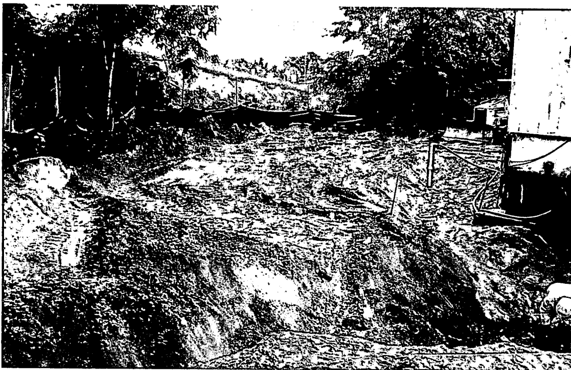
View of southern cell after backfill has been placed.
