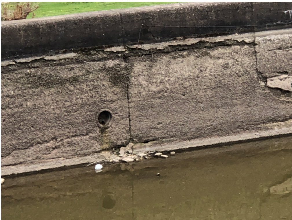
NYS Canal Corp. Wall Drainage Piping – Looking south
