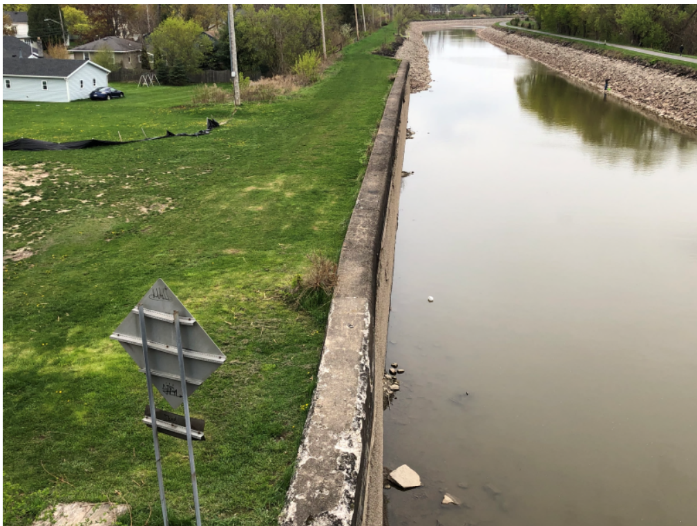
NYS Canal Corporation Wall – Looking west
