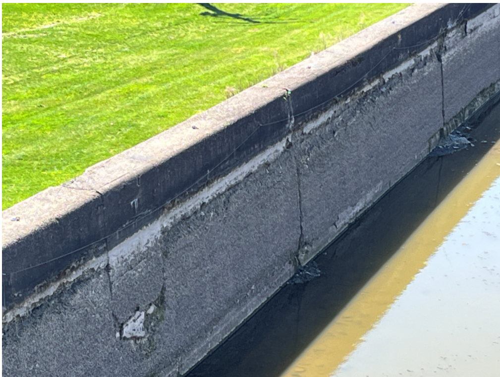
Central portion of NYS Canal Corporation Wall- Looking southwest
