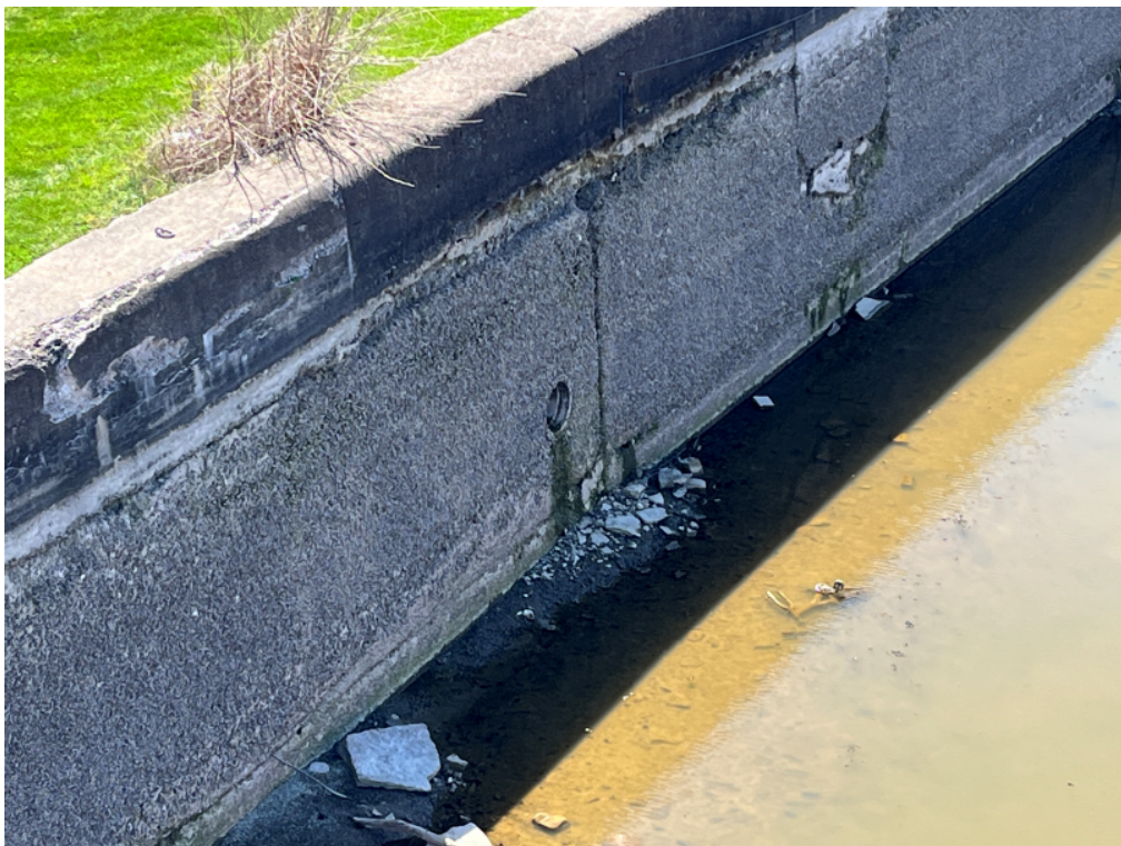
NYS Canal Corp. Wall Drainage Piping – Looking southwest
