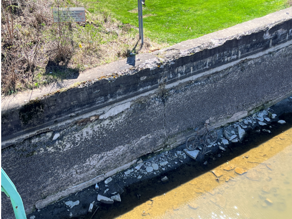
East portion of NYS Canal Corporation Wall- Looking southwest
