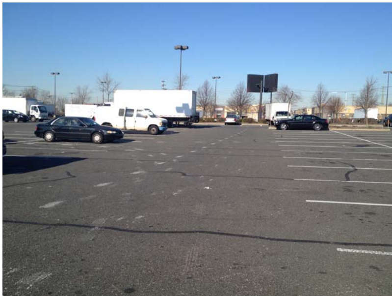
Photo #15: A view of the asphalt covered parking lot and repaired cracks on the eastern side of the parking lot. View is to the north.
