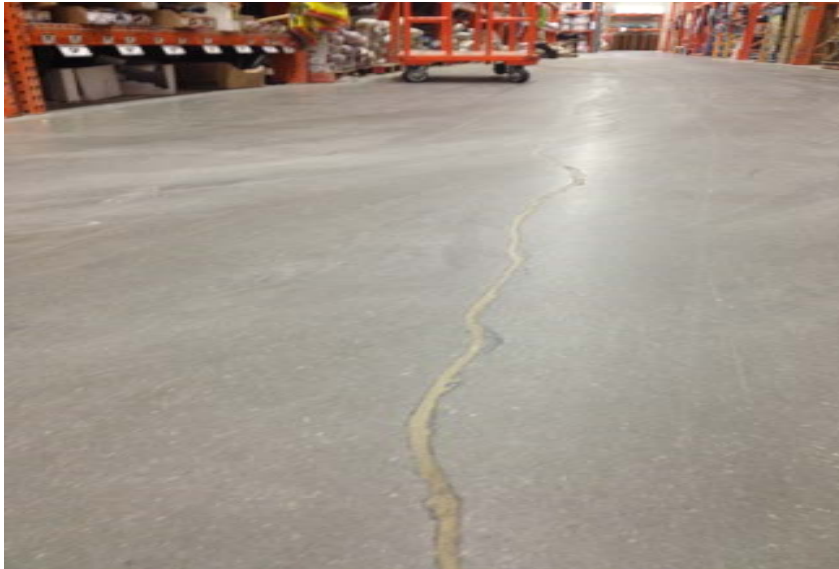
Photo #1: A view of the concrete building slab and repaired crack on the western side of the building. View is to the south.
