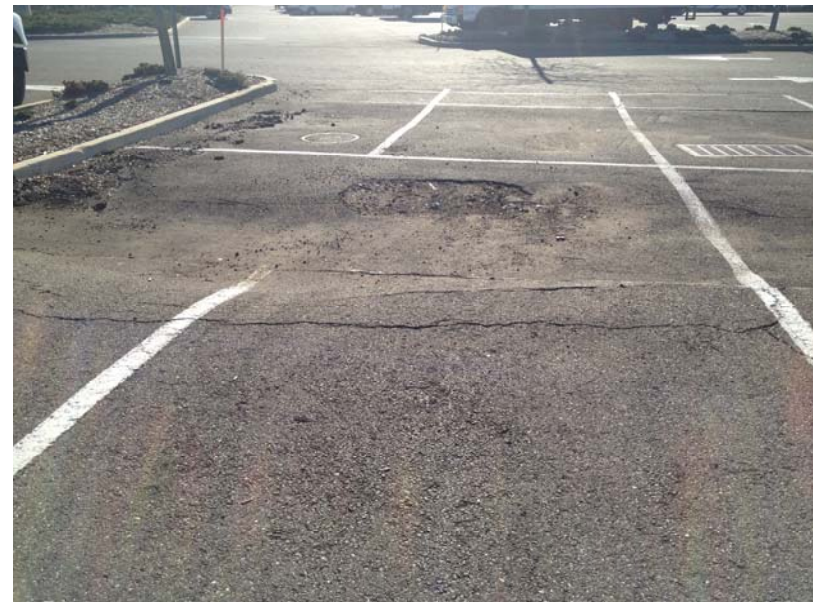
Photo #17: A view of asphalt buckling on the northern portion of the parking lot. View is to the south.
