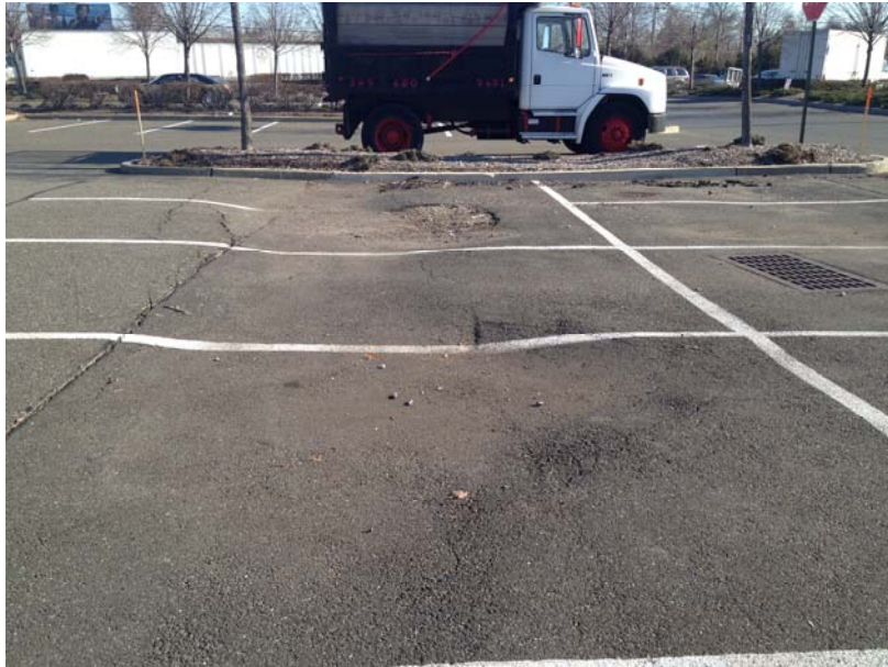
Photo #18: A view of asphalt buckling on the northern portion of the parking lot. View is to the east.
