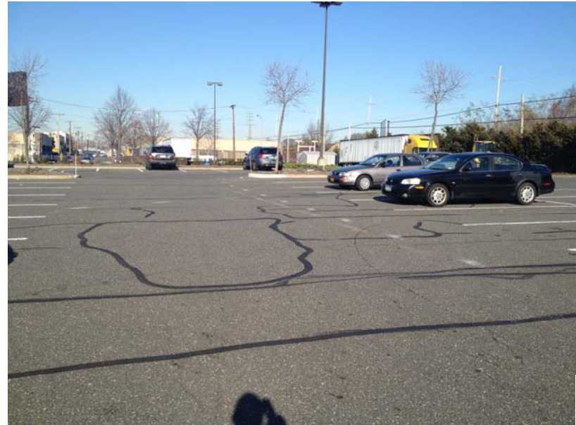
Photo #14: A view of the asphalt covered parking lot and repaired cracks on the eastern side of the parking lot. View is to the north.
