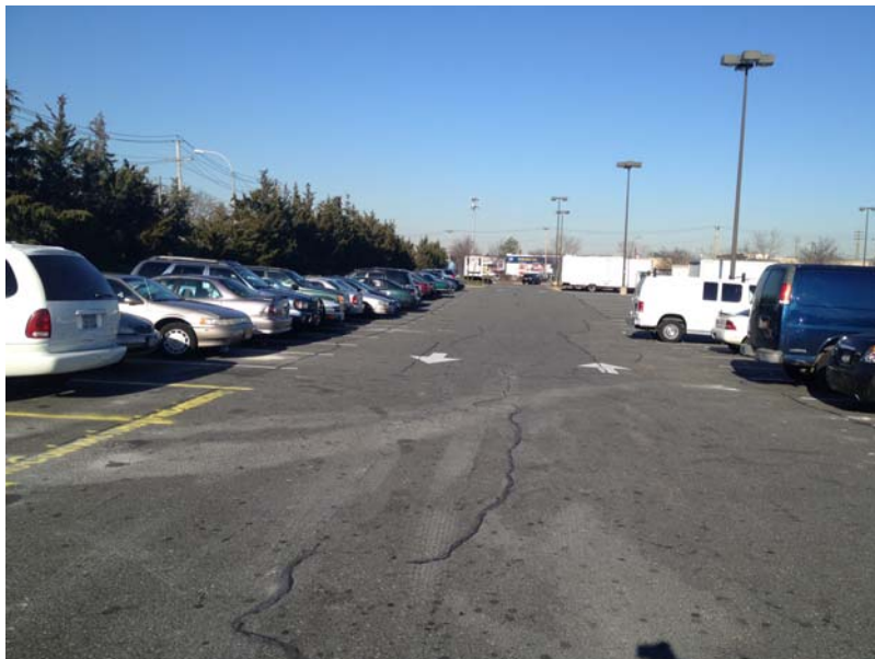
Photo #11: A view of the asphalt covered parking lot and repaired cracks on the western side of the parking lot. View is to the north.
