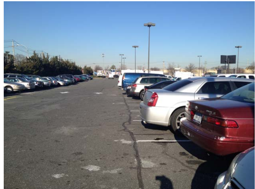
Photo #10: A view of the asphalt covered parking lot and repaired cracks on the western side of the parking lot. View is to the north.
