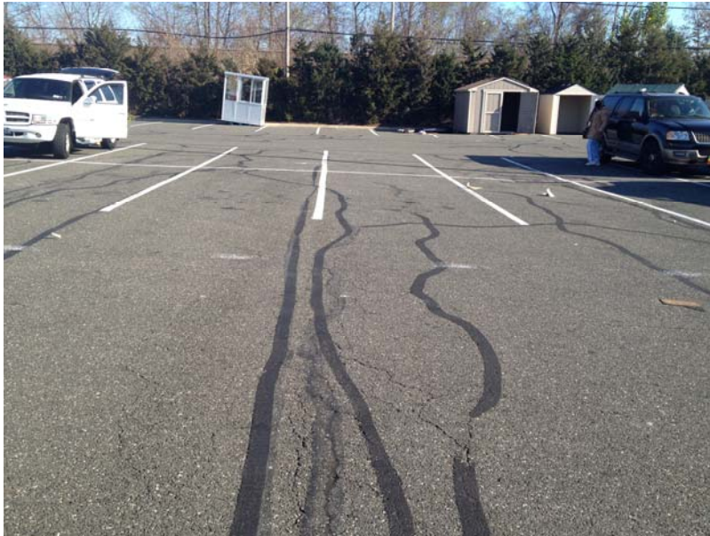
Photo #13: A view of the asphalt covered parking lot and repaired cracks on the eastern side of the parking lot. View is to the east.
