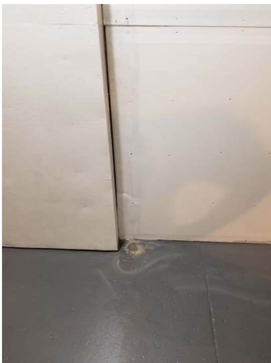
PHOTO 3 & 4: PATCHED FLOOR PENETRATION (REMOVED EXTRACTION POINT) & CAPPED LATERAL PIPING
