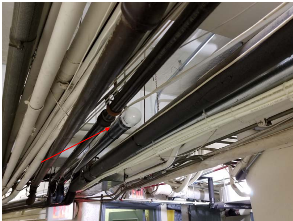
PHOTO 4: CAPPED LATERAL PIPING
