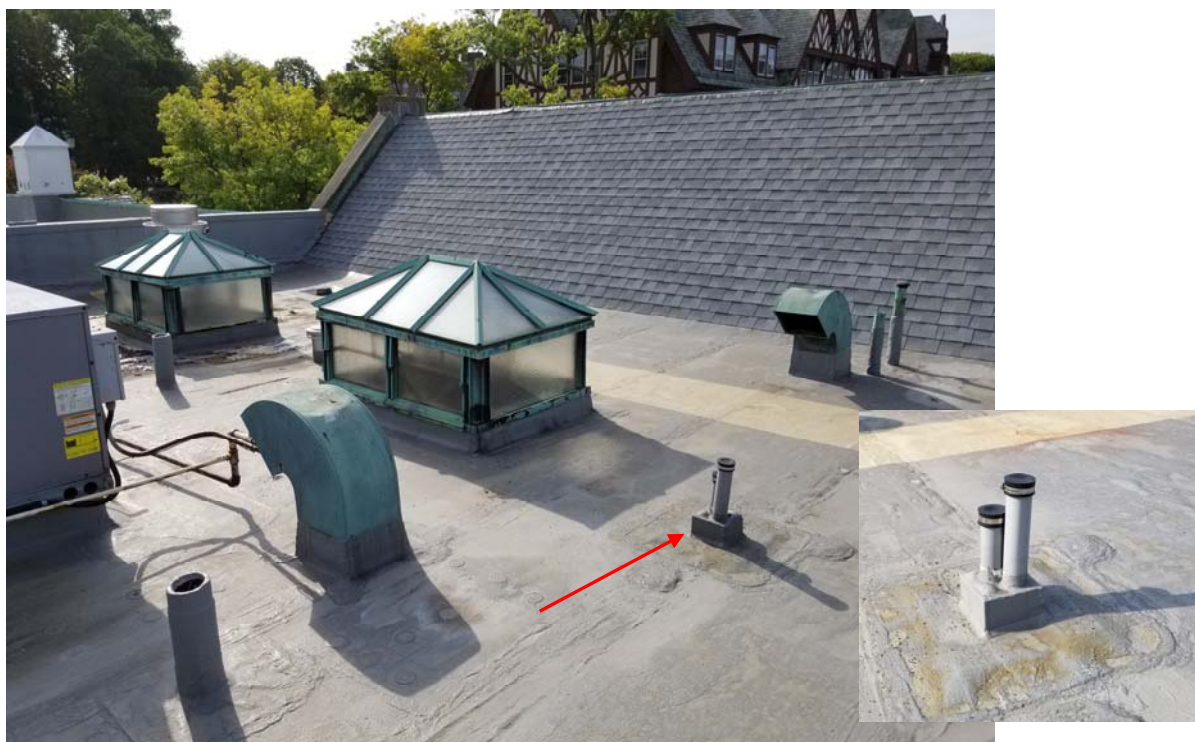
PHOTO 6: ROOF PENETRATION PIPING CUT & CAPPED (ROOFER WILL CUT PIPES & RESEAL PENETRATION)
