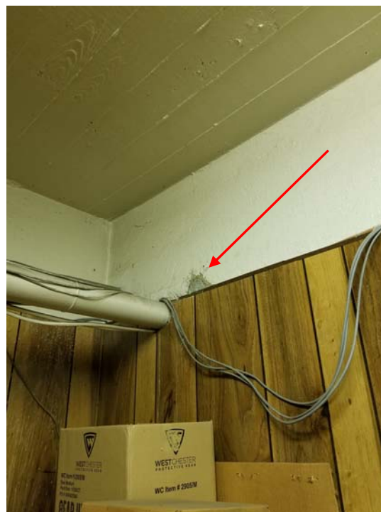
PHOTO 2: EXTRACTION PIPE CUT, GROUTED & CAPPED.
