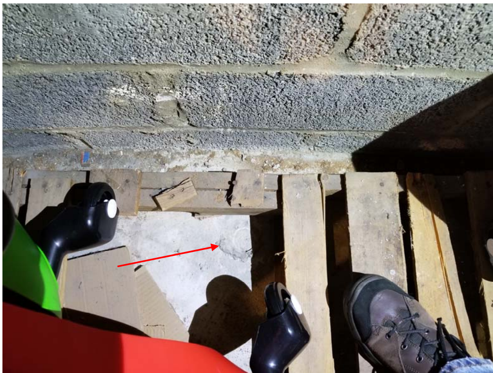
PHOTO 3: PATCHED FLOOR PENETRATION (SEALED EXTRACTION POINT)
