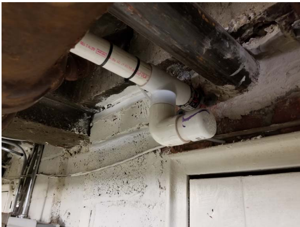
PHOTO 2: CAPPED LATERAL PIPING
