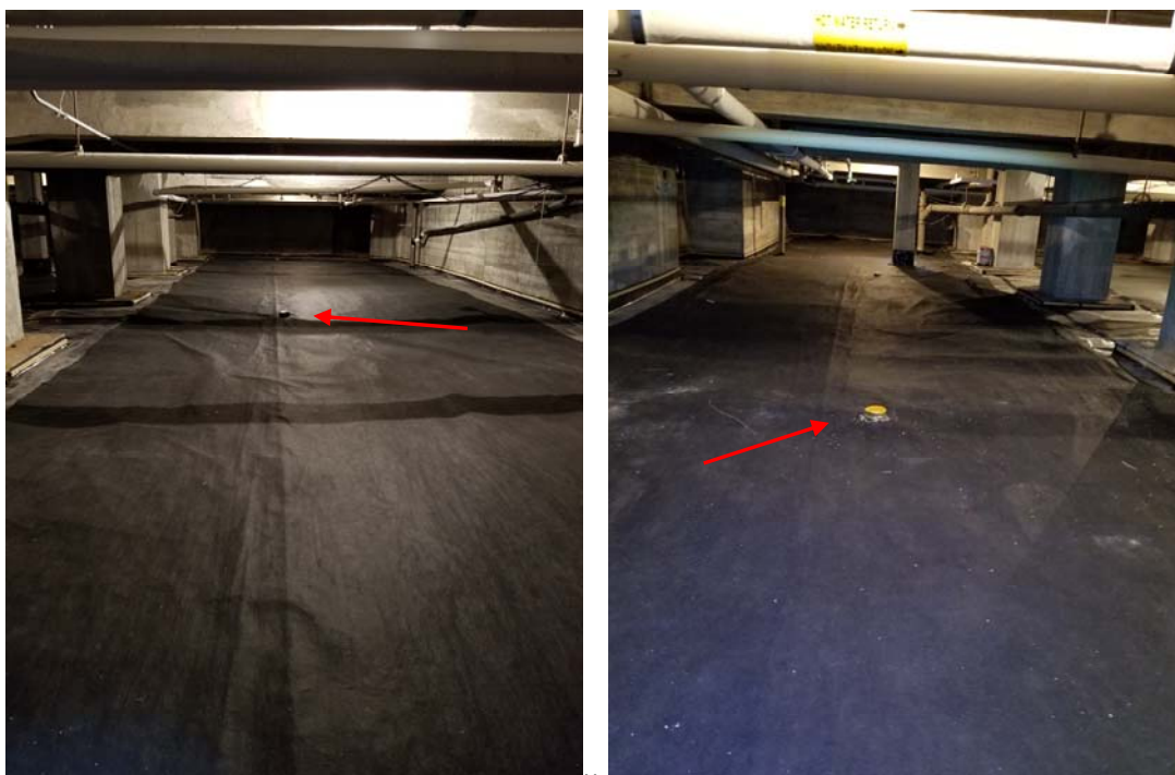
PHOTO 6 & 7: GEO-MEMBRANE LEFT IN PLACE IN EASTERN PORTION OF BASEMENT. EXTRACTION POINTS IN THIS AREA WERE CUT, GROUTED & CAPPED.
