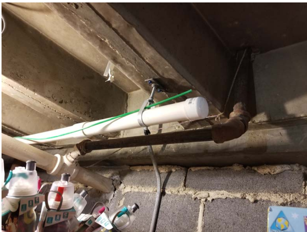
PHOTO 4: CAPPED LATERAL PIPING
