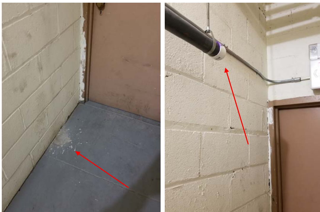
PHOTO 7 & 8: PATCHED FLOOR PENETRATION (REMOVED EXTRACTION POINT) & CAPPED LATERAL PIPING
