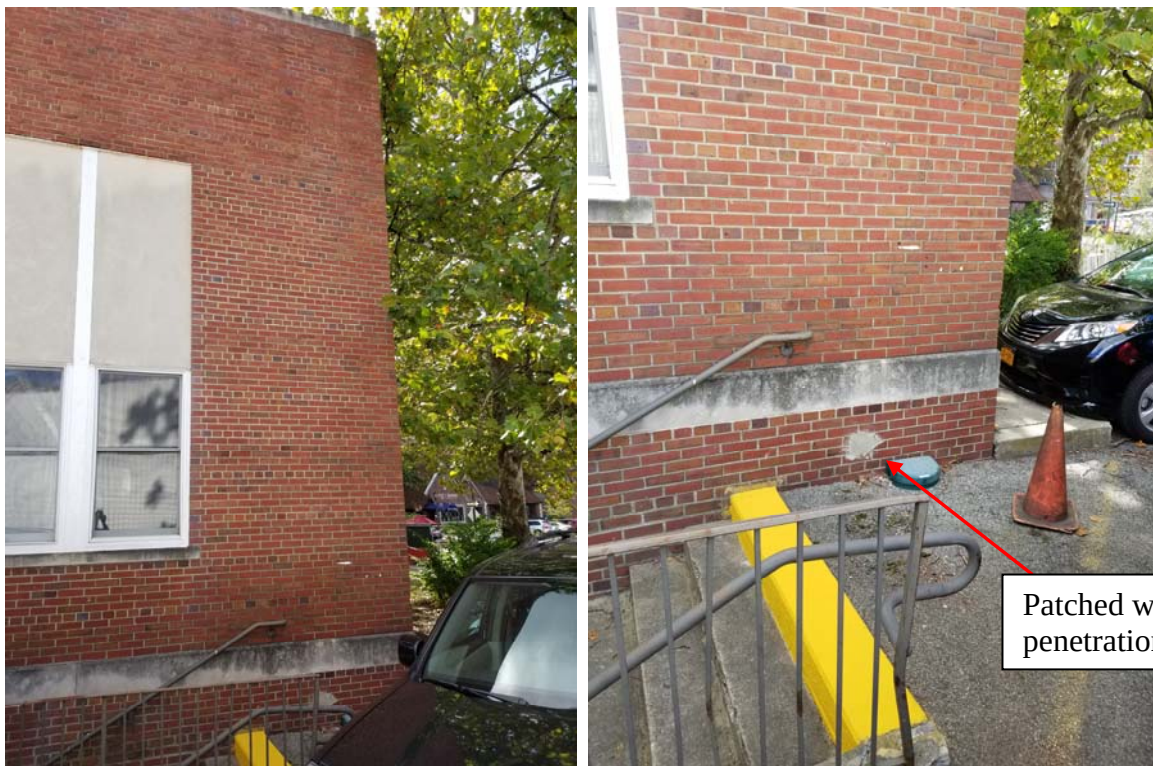
PHOTO 9 & 10: DISCHARGE PIPE RUNNING UP TO BLOWER ON ROOF REMOVED. THROUGH WALL PENETRATION PATCHED.
