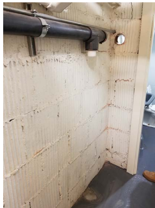
PHOTO 3 & 4: PATCHED FLOOR PENETRATION (REMOVED EXTRACTION POINT) & CAPPED LATERAL PIPING
