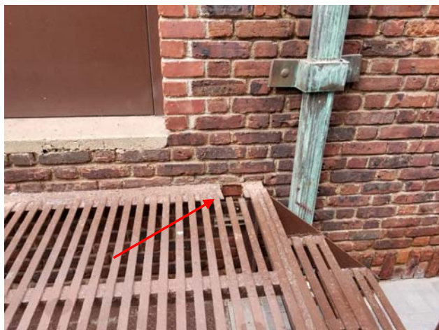
PHOTO 9 & 10: DISCHARGE PIPE REMOVED FROM WALL & HOLE WHERE DISCHARGE PIPE WHEN THROUGH LANDING
