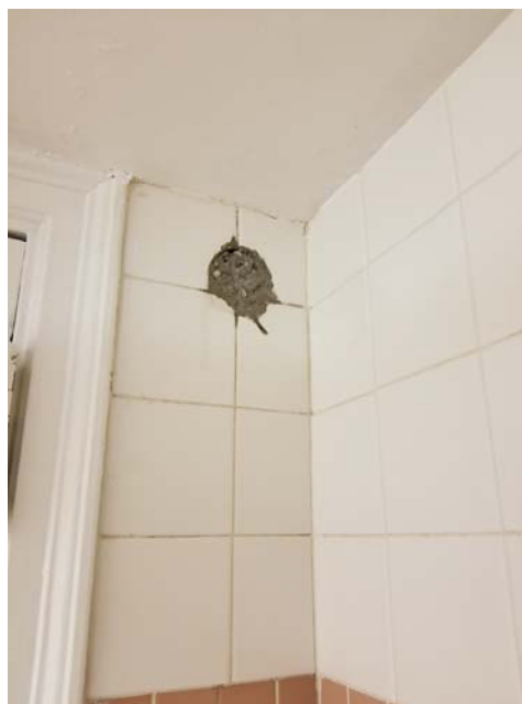
PHOTO 2 & 3: PATCHED FLOOR & WALL PENETRATION (REMOVED EXTRACTION POINT)
