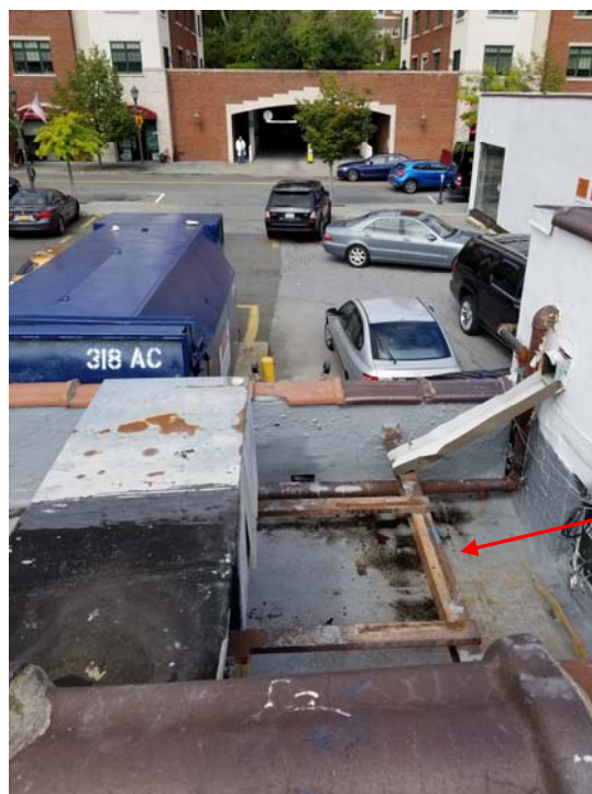
PHOTO 7: REMOVED BLOWER & HOUSING
