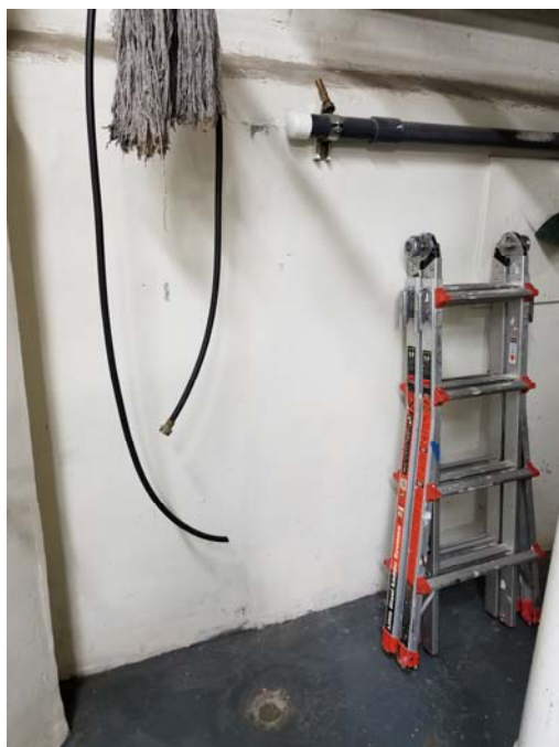
PHOTO 5 & 6: PATCHED FLOOR PENETRATION (REMOVED EXTRACTION POINTS) & CAPPED LATERAL PIPING
