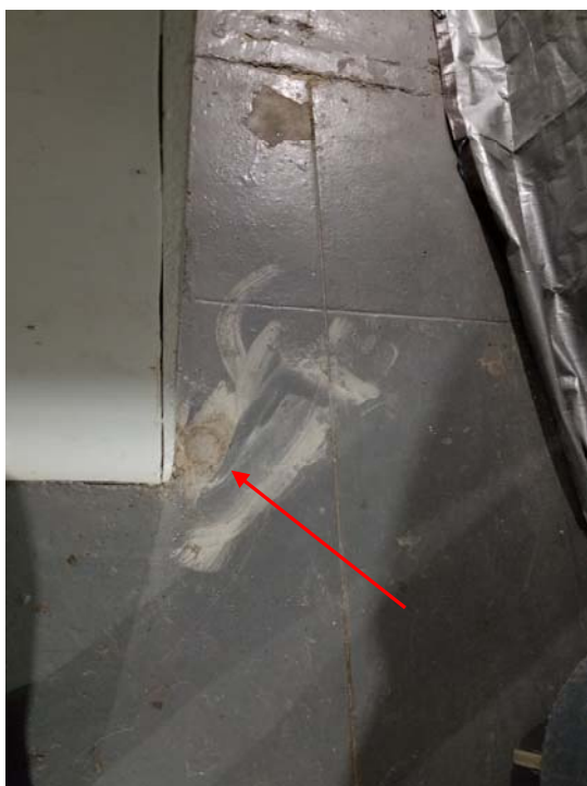
PHOTO 1 & 2: PATCHED FLOOR PENETRATION (REMOVED EXTRACTION POINT) & CAPPED LATERAL PIPING (NORTH END AREA)
