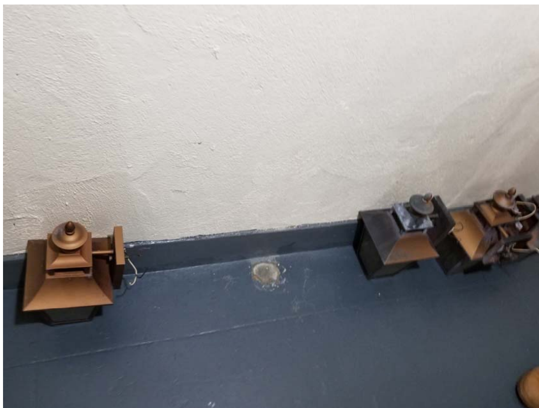
PHOTO 1: PATCHED FLOOR PENETRATION (REMOVED EXTRACTION POINT)
