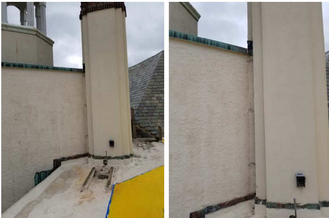
PHOTO 8 & 9: REMOVED BLOWER & HOUSING & DISCHARGE PIPE
