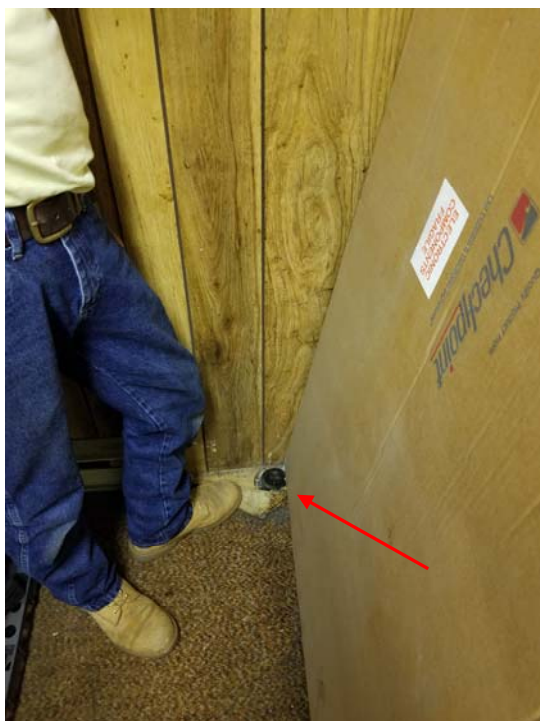
PHOTO 2: EXTRACTION PIPE CUT, GROUTED & CAPPED.
