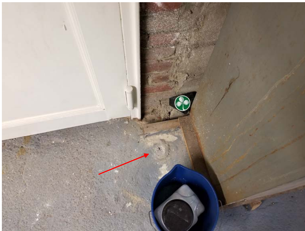
PHOTO 1: PATCHED FLOOR PENETRATION (REMOVED EXTRACTION POINT)
