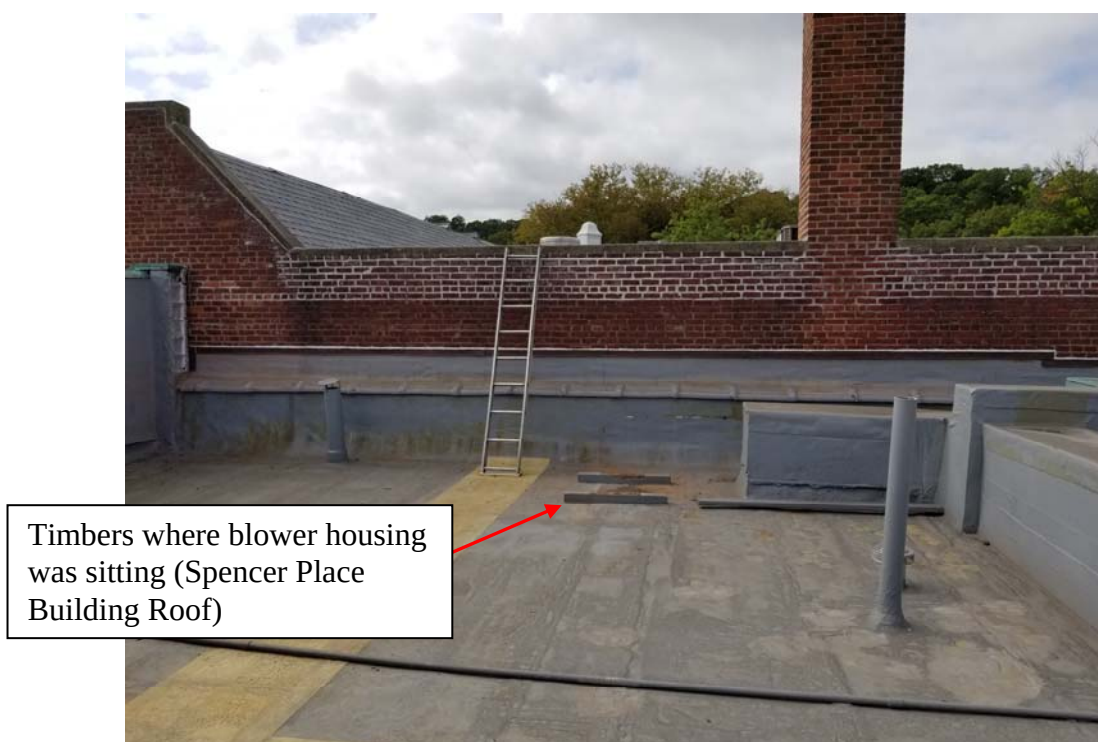
PHOTO 7: REMOVED BLOWER & HOUSING
