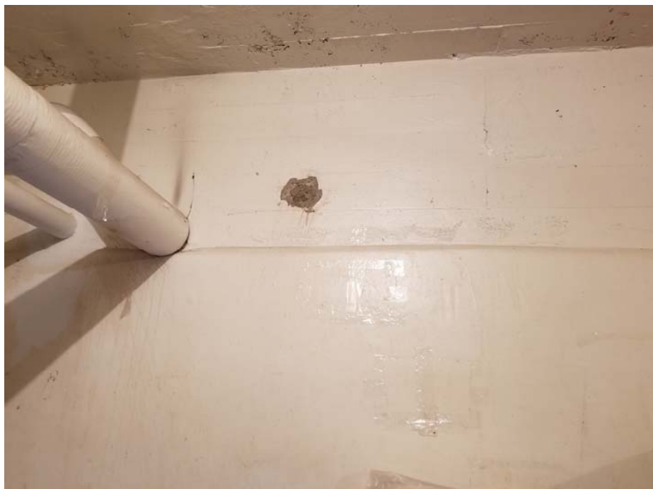
PHOTO 5: LATERAL PIPING REMOVED & THROUGH WALL PENETRATIONS PATCHED.
