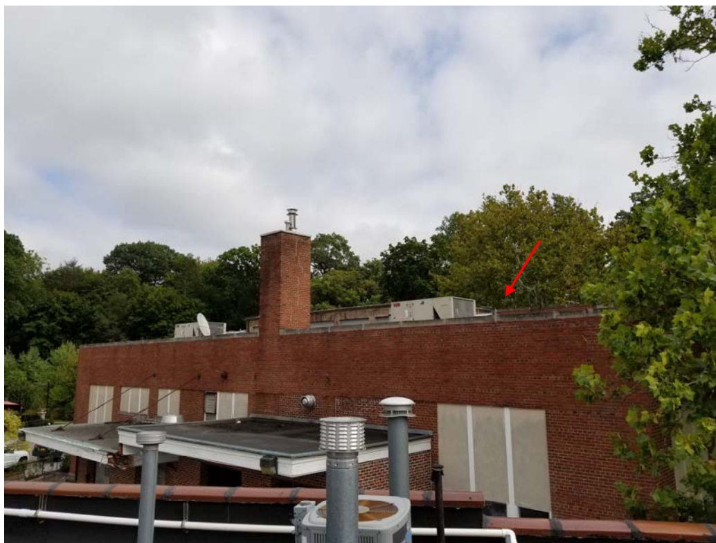
PHOTO 11: BLOWER & BLOWER HOUSING ON ROOF REMOVED.
