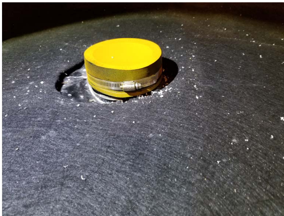
PHOTO 8: CLOSE-UP OF CUT, GROUTED & CAPPED EXTRACTION POINT IN EASTERN PORTION OF BASEMENT.
