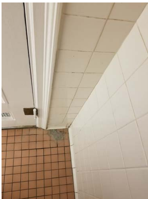
PHOTO 2 & 3: PATCHED FLOOR & WALL PENETRATION (REMOVED EXTRACTION POINT)
