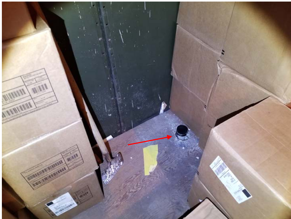
PHOTO 4: CUT, GROUTED & CAPPED EXTRACTION POINT IN AREA OF RAISED FLOOR.
