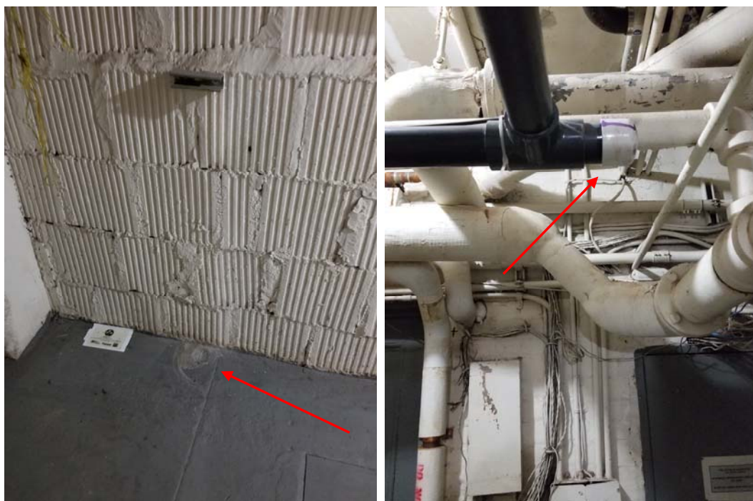
PHOTO 5 & 6: PATCHED FLOOR PENETRATION (REMOVED EXTRACTION POINT) & CAPPED LATERAL PIPING
