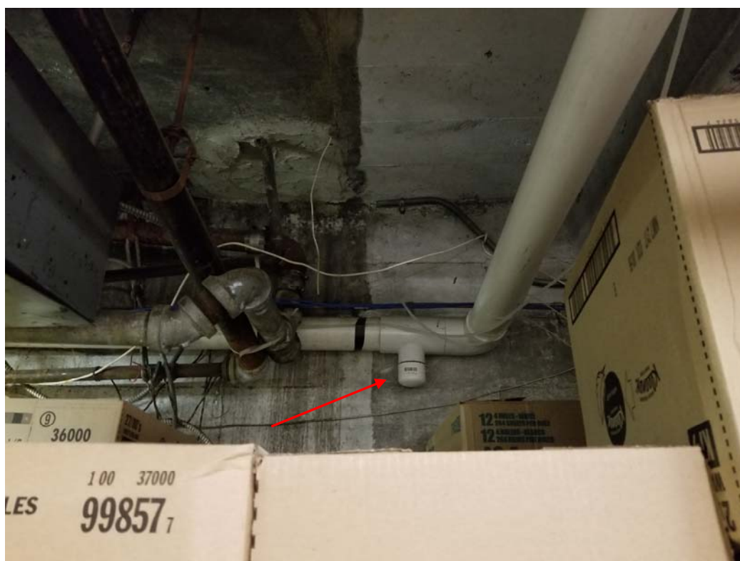
PHOTO 3: EXTRACTION PIPE REMOVED AND CUT & CAPPED
