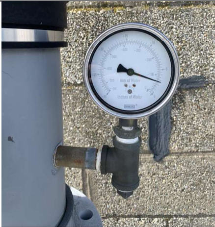
Photo 10: Suction Fan Vacuum Gauge at VR-1.
