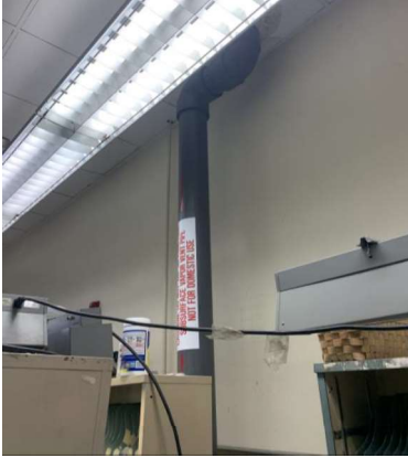
Photo 1: Sub-Slab Depressurization System (SSDS) Riser, VR-1.
