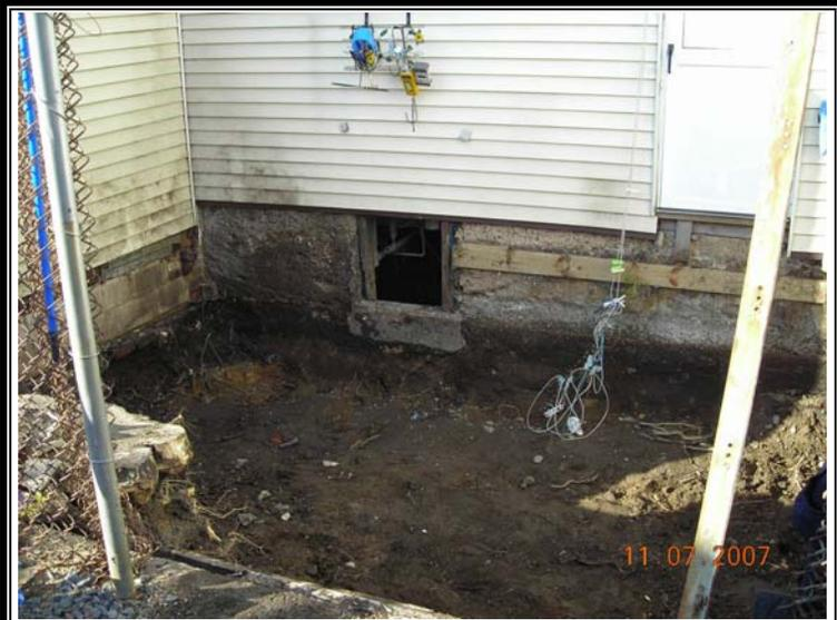
**Photo 1** – View of 57-42 after using Vactron to remove top one foot of soil in November 2008.
