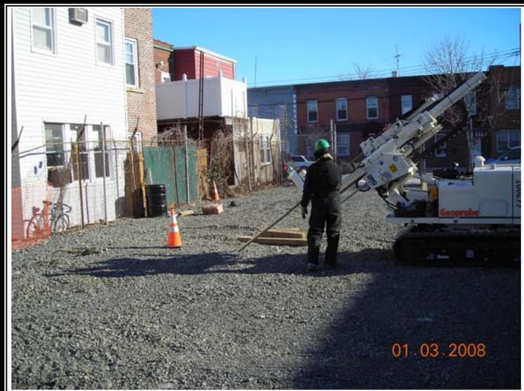
**Photo 4** – View of Geoprobe advancing sampler under fence footer, into backyard of 57-42 in January 2008.
