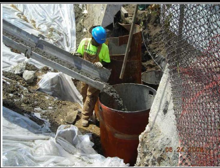
**Photo 9** – Pouring of concrete into excavated cans in 57-42 backyard in June 2008.
