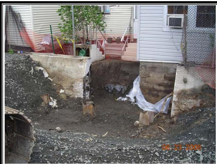
**Photo 5** – View of 57-42 backyard with fence footer removed, previously installed clean fill removed, ready to begin installation of overdrill cans in June 2008.
