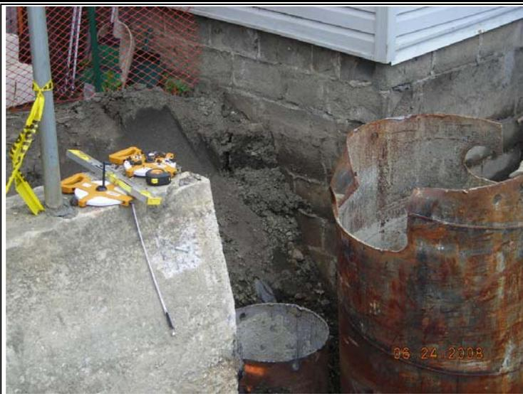
**Photo 8** – Excavated cans in backyard of 57-42, ready for concrete pour, June 2008.
