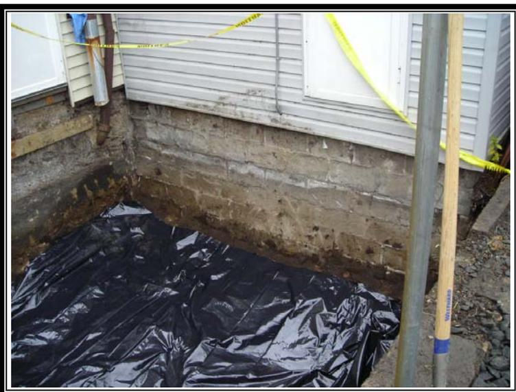
**Photo 3** – View of 57-52 post excavation showing plastic liner installed prior to back-filling.
