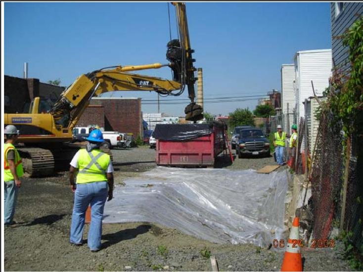
**Photo 7** – Disposal of soil from overdrill behind 57-42 into on-site container.
