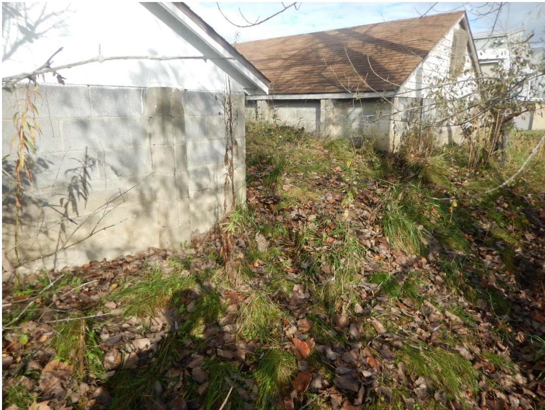
Photo 10: Taken November 1, 2022. AOC-4: Conditions generally acceptable. Shallow rodent burrows present along building edge (patched by RM management prior to LaBella inspection).
