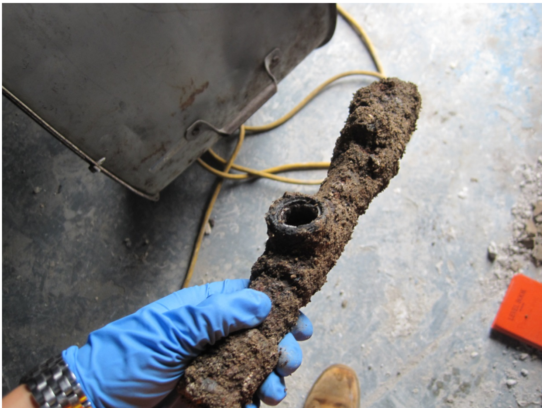
Photo 2: Section of piping unearthed during excavation of test pit TPD-1.
