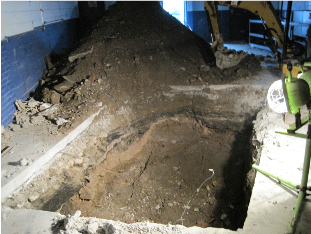
Photo 1: Test pit TPD-1.
