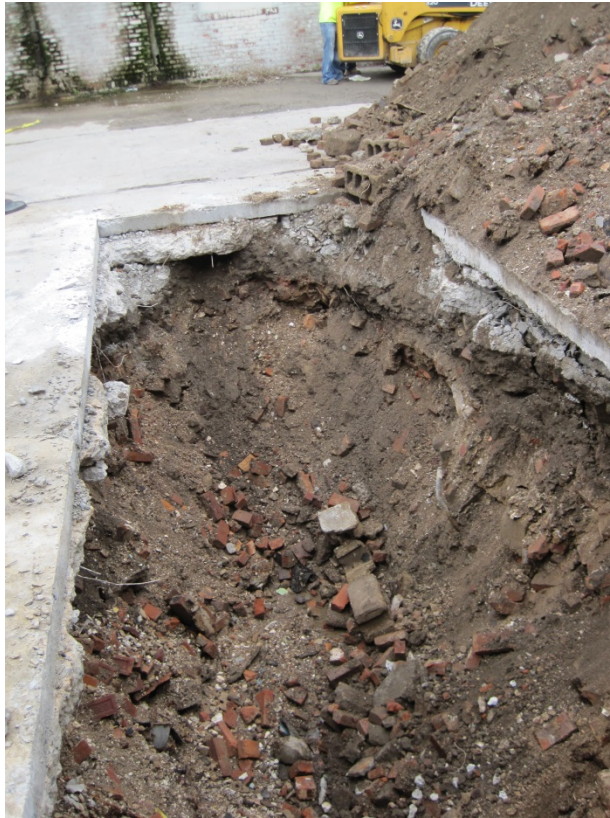
Photo 7: View of test pit TPD-3 perpendicular to Building 25A.
