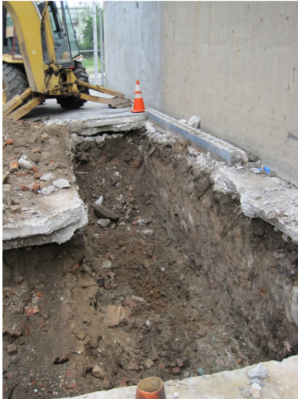
Photo 5: View of test pit TPD-3 parallel and adjacent to Building 25A.
