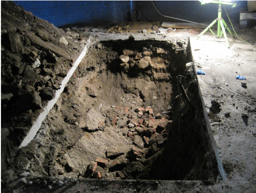
Photo 3: Test pit TPD-2.
