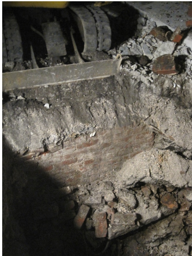
Photo 4: Intact brick wall in test pit TPD-2.
