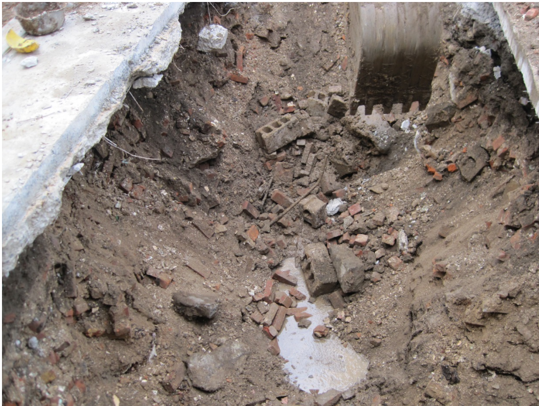
Photo 8: Excavated materials in portion of test pit TPD-3 perpendicular to Building 25A.
