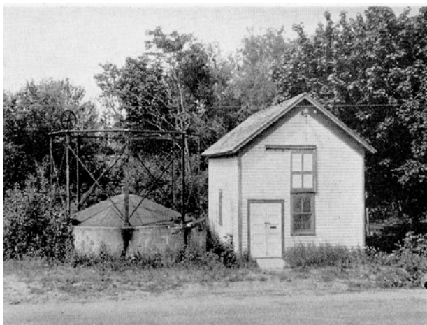
Southold—Acetylene Gas Plant
