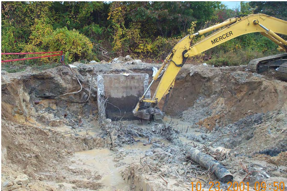
View looking east at demolition of East Drip Pit
