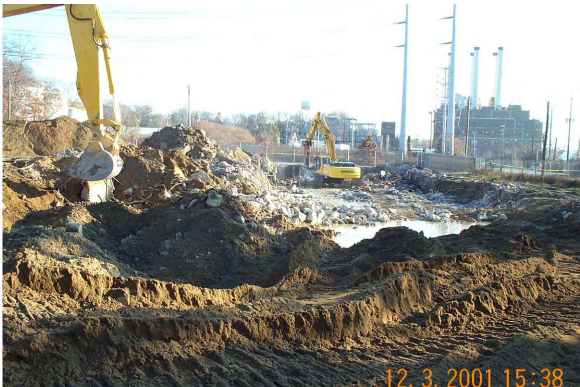
View looking south at comp. bldg. demo and backfilling
