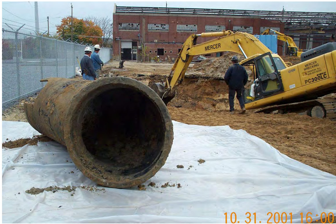
View looking west at abandoned 45" da. Cast iron gas main from vicinity of south drip pit excavation
