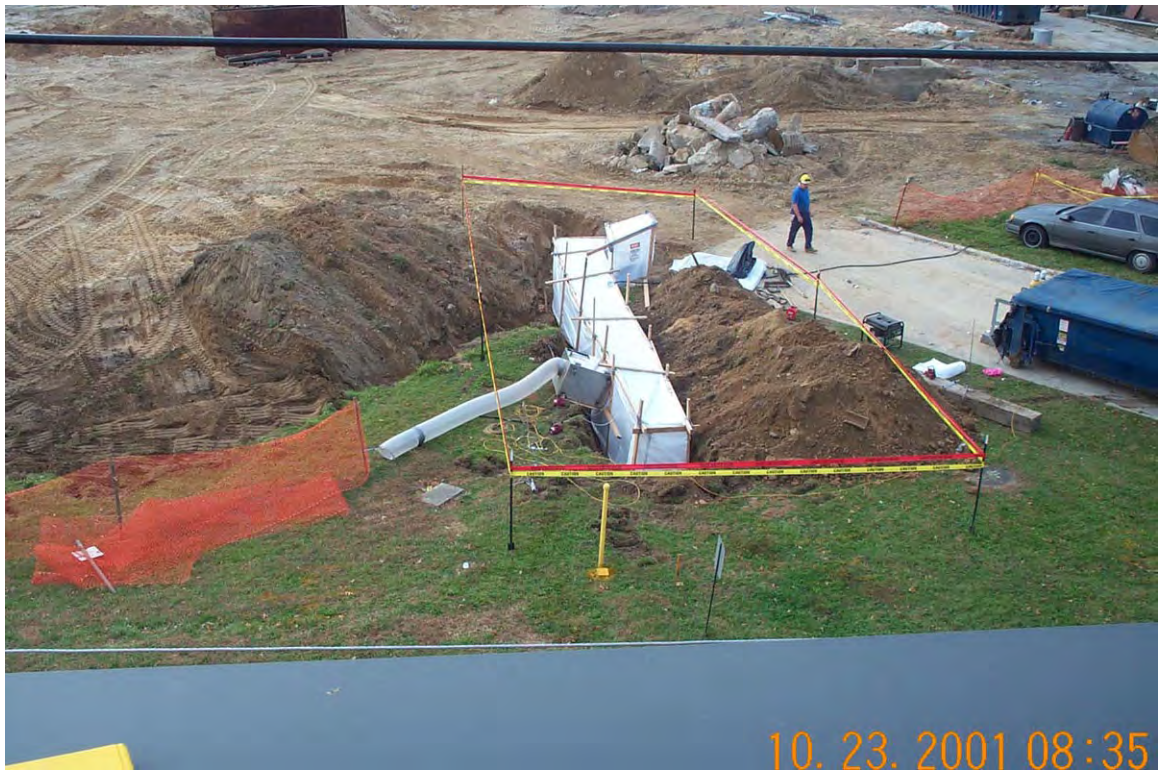
Asbestos enclosure constructed over drip line for abatement - View south from lab roof
