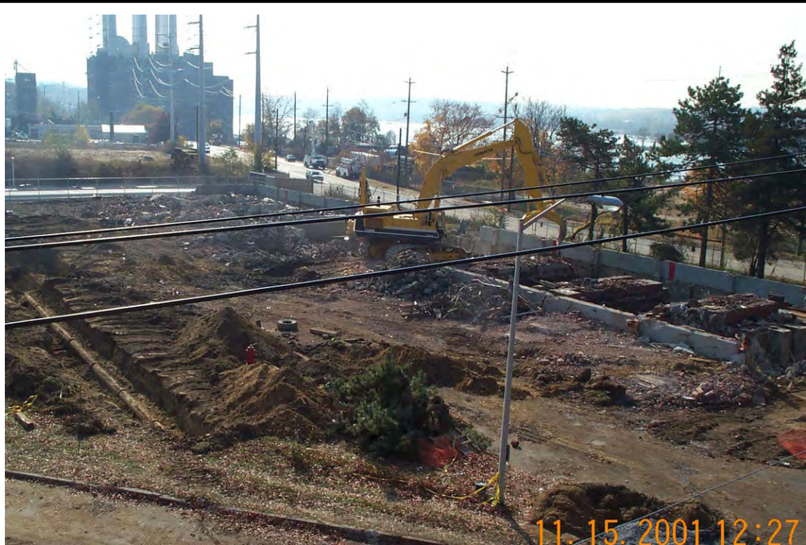
View looking southwest at grapple and hoeram during demo of comp. bldg. foundation
