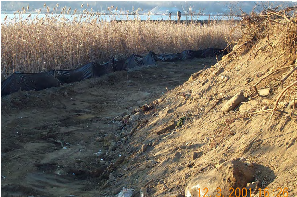
View looking northwest at slope preparation for rip rap along edge of area 1B
