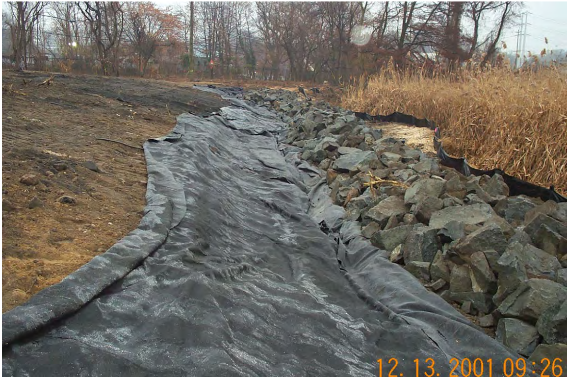
View looking southeast at geotextile and rip rap placements in area 1B
