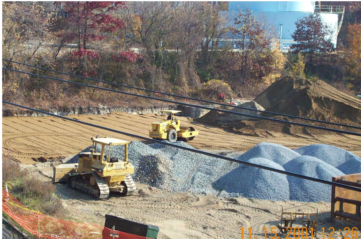
View looking southeast of area 3-1 at sand backfill compaction
