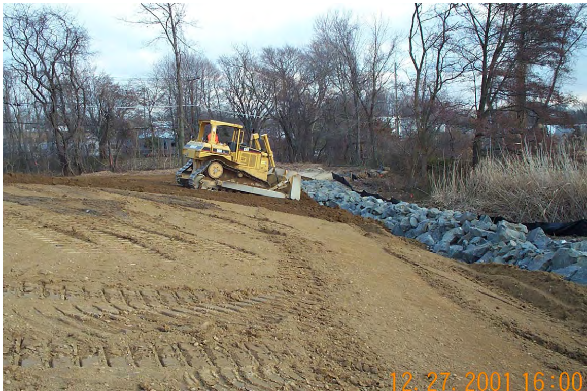
View looking southeast at dozer spreading clay soils in area 1B
