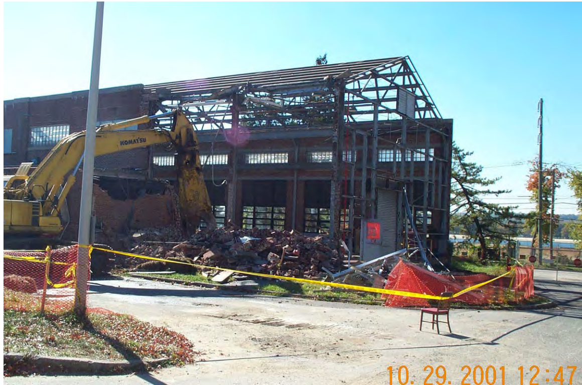
View looking southwest at beginning of demolition of compressor building. Brick facade is being stripped off of structural steel
