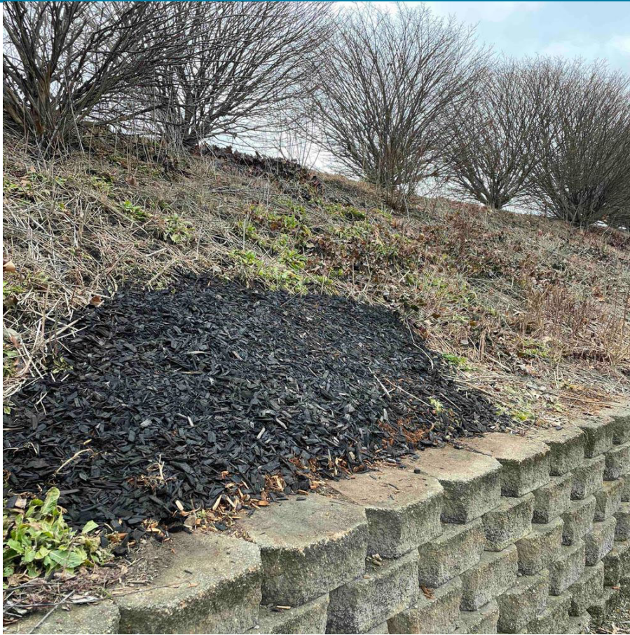
Photo 3: Animal burrow backfilled and area covered with mulch. Photograph taken 2-17-2023.
