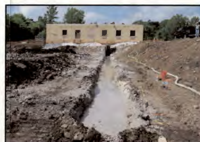
CB Slurry Wall Area 1
