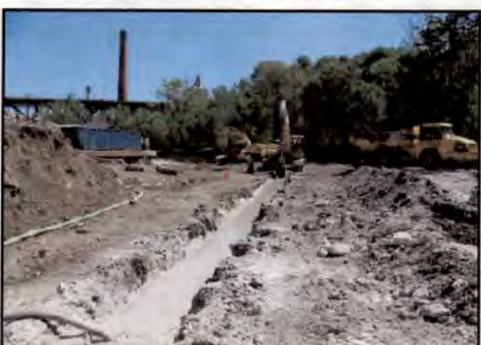
CB Slurry Wall Area 1
