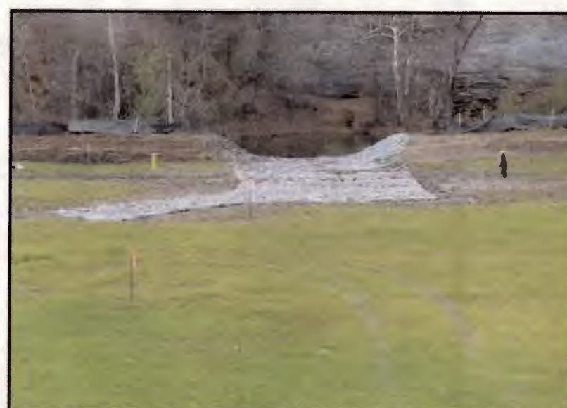
Completed Swale and Berm Cut-Out (11-12-08)
