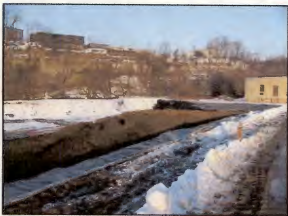
BACKFILL OF AREA 1 WITH AREA 3 MATERIAL
