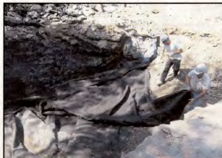
Geotextile Over Pea Gravel in Southern Channe
