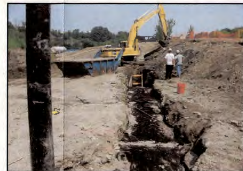
Collection Trench with Geotextile Over Gravel
