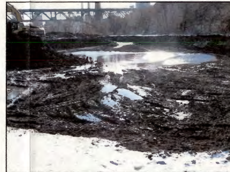
REMOVAL OF MATERIAL TO FINAL EXCAVATION DEPTH BELOW WATER TABLE (390' - 391') IN AREA 1
