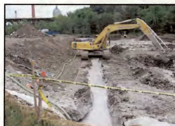
CB Slurry Wall Area 1
