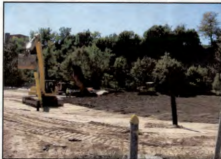
Grading and Restoration Activities Area 1 (9-2-08) (Topsoil Over Imported Fill)
