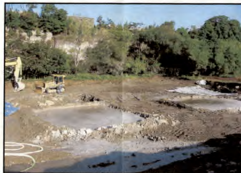
Spoil Mixing Pits in Area 1
