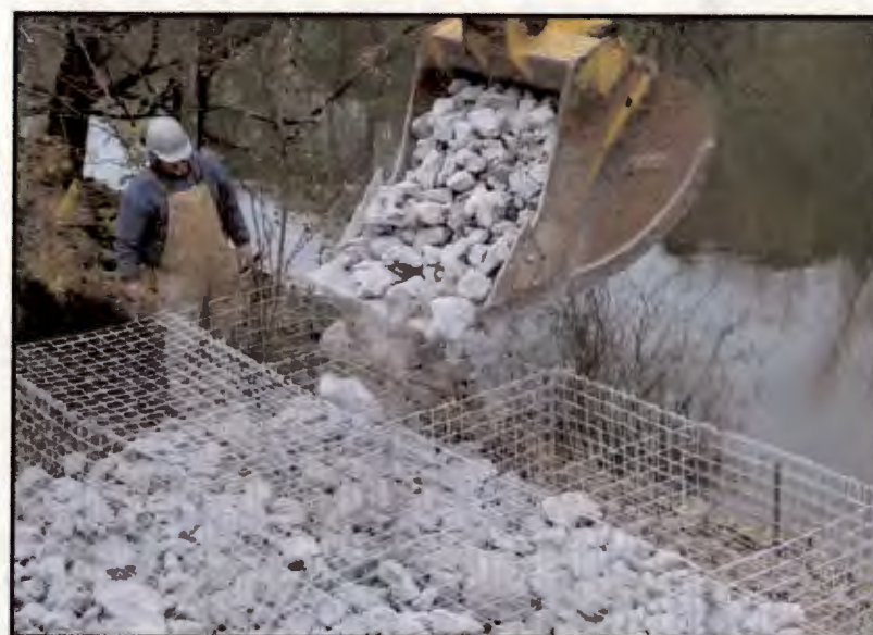
Gabion Construction
