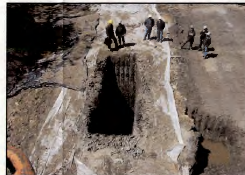
Test Pit at Columns B-6, B-7 and B-8 (5-28-08) Showing Water Level East of ISS Barrier
