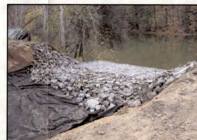
Riprap Placement (Lower End)
