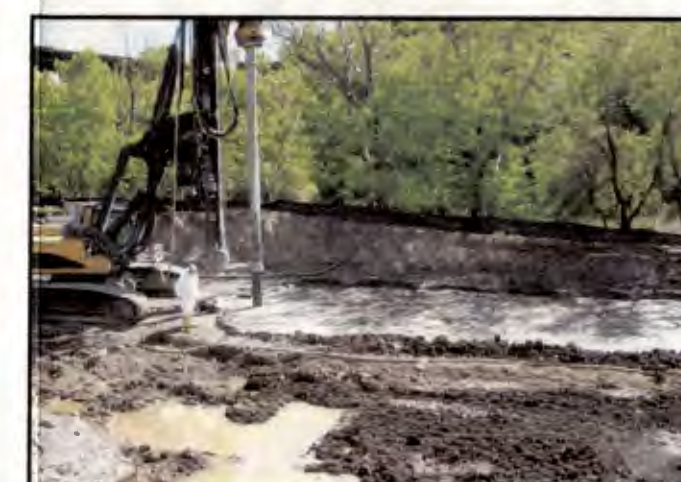
ISS Column Construction Area 1
