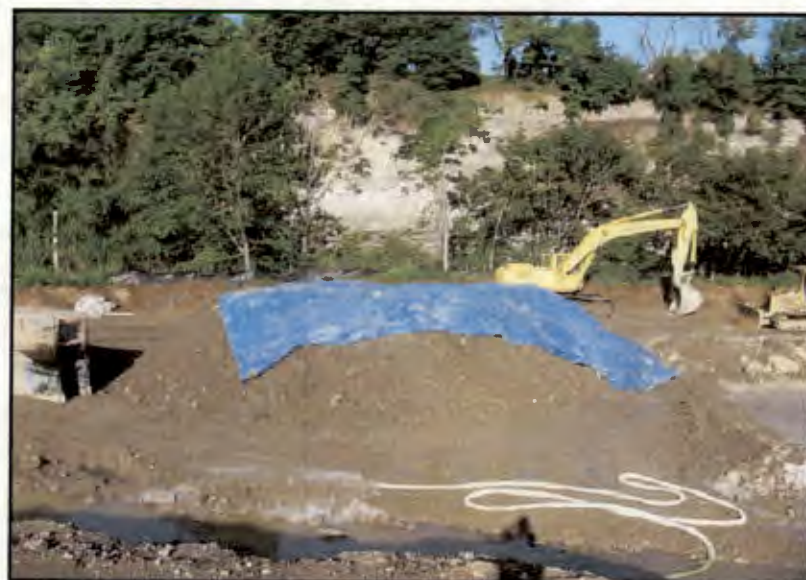
Stabilized Spoils Stockpile in Area 1
