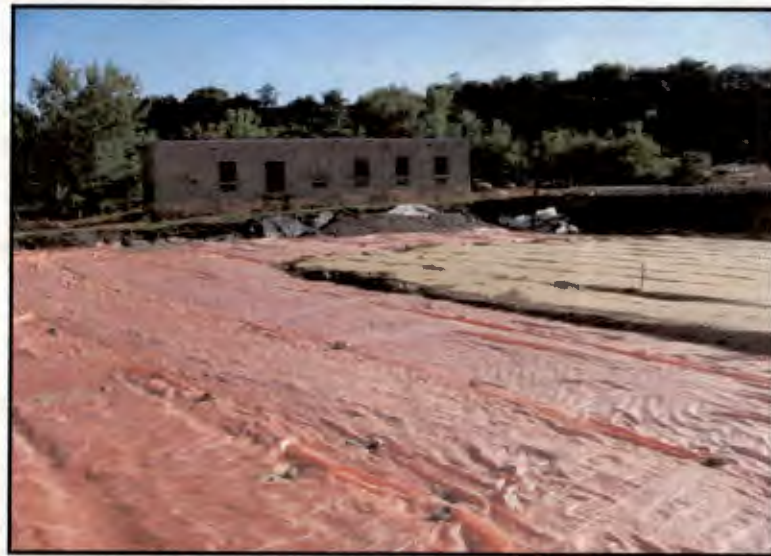
Grading and Restoration Activities Area 1 (8-26-08) (Showing Orange Delineation Fabric Installation)
