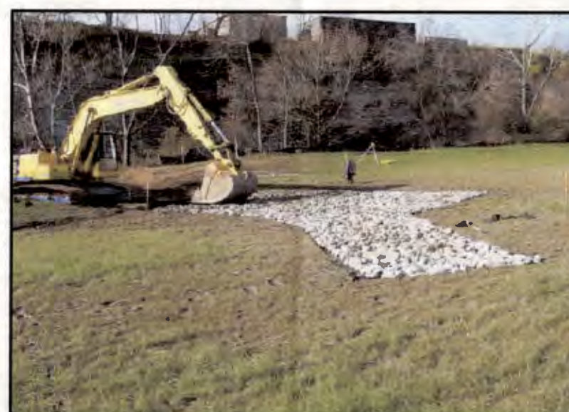
Riprap Placement (Upper End)
