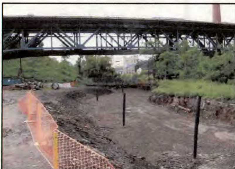
Collection Trench Following Backfill over Fabric
