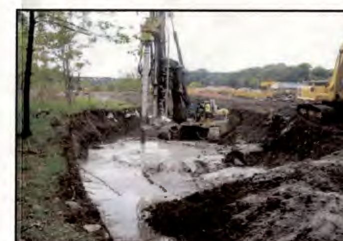
ISS Column Construction Area 3
