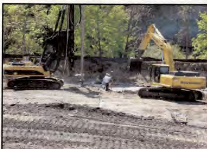
ISS Column Construction Area 2 and Excavator for Swell Management and Obstruction Removal
