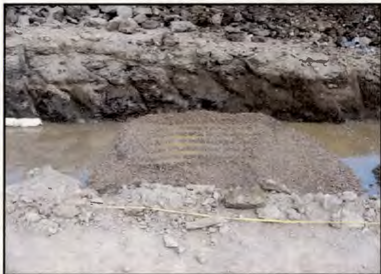
Pea Gravel Placement in Northern Channel
