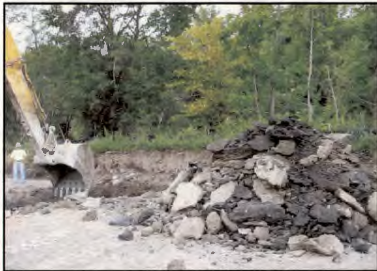
Removing Stabilized Material in Northern Channel
