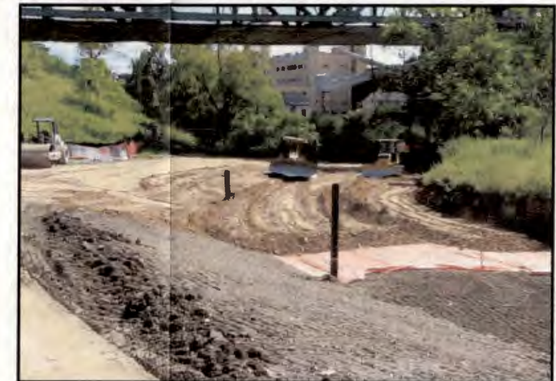
Grading and Restoration Activities Area 3 (8-19-08) (Showing Backfill Over Delineation Fabric)
