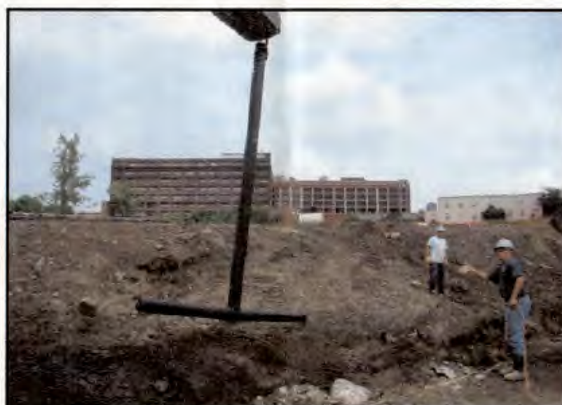
Vertical Recovery Point Construction and Placement
