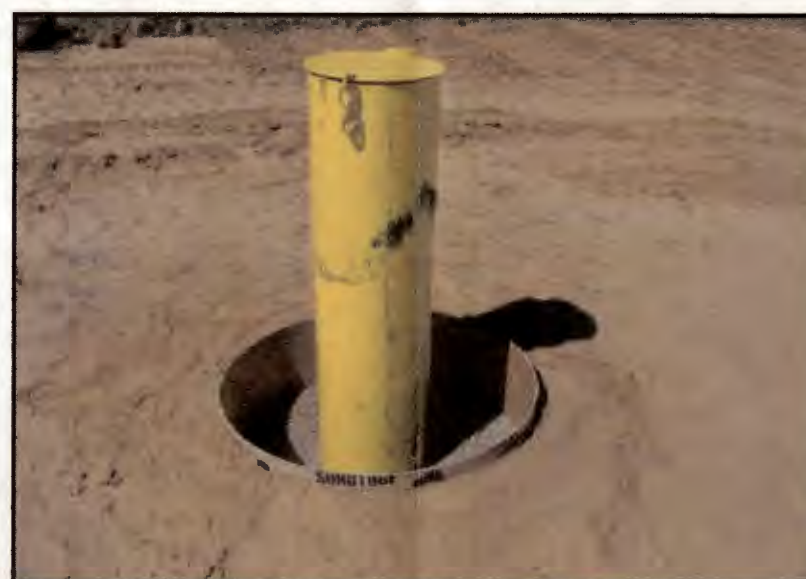
Recovery Well Casing and Sonotube
