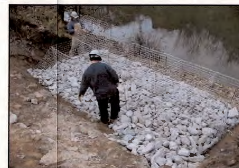
Gabion Construction
