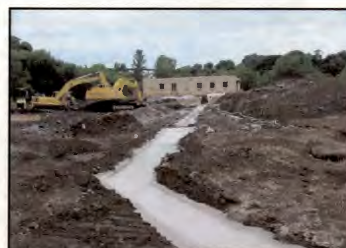
CB Slurry Wall Area 1
