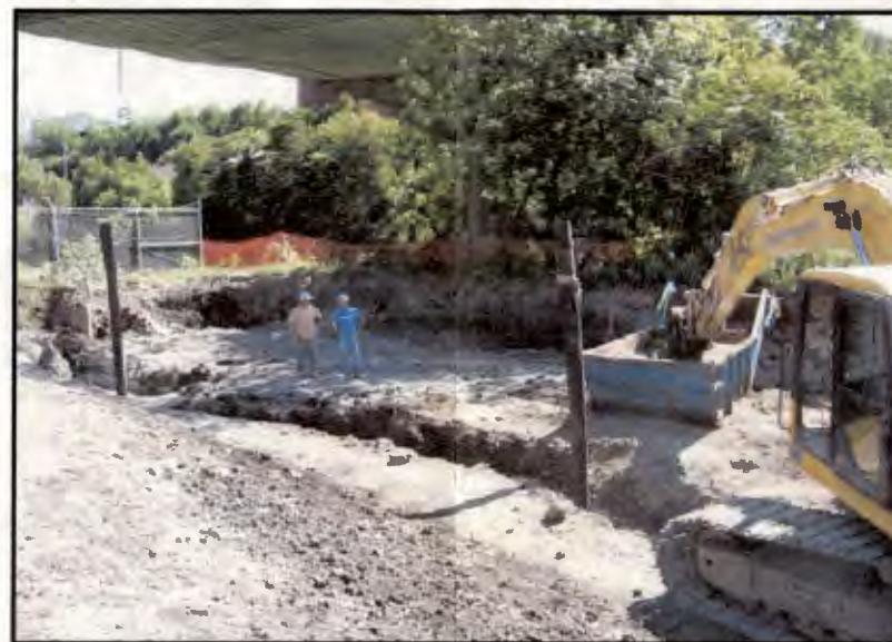
Collection Trench Construction
