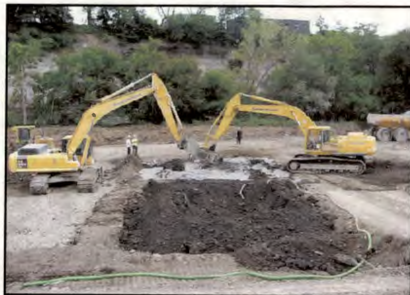
Spoils Mixing in Cell in Area 1
