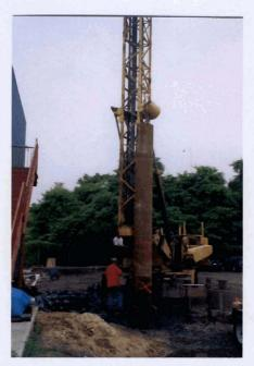
4. Installation of DNAPL/LNAPL Removal Monitoring System auger casing installation.
