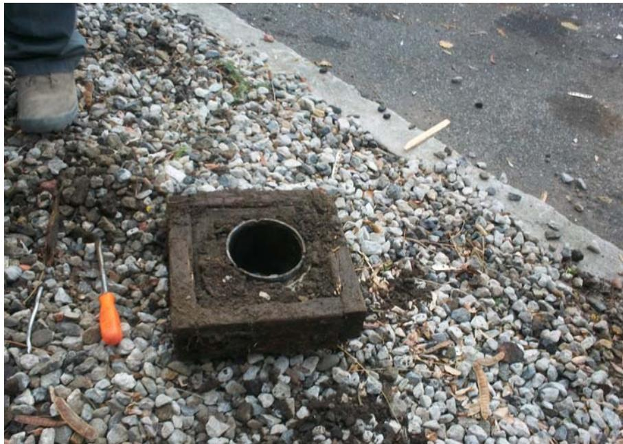
2. Detached well casing of monitoring well MW-3, located in the northeastern corner of the Site, on December 3, 2013.
