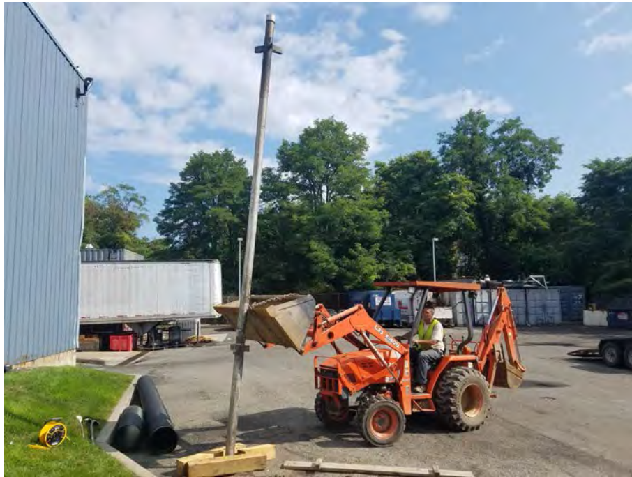
5. Removal of 4-inch diameter recovery pipe of the DNAPL recovery well
