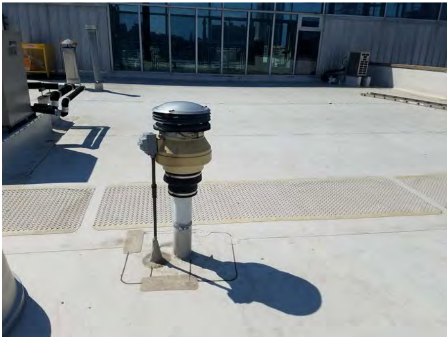
4. One of four active rooftop fan units for vapor mitigation system
