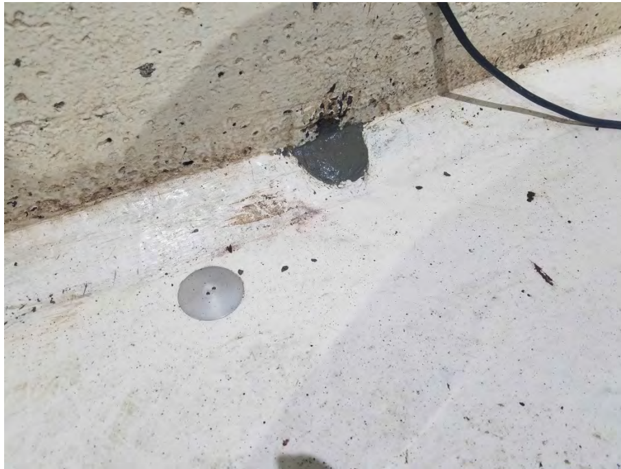
9. New VES monitoring point and old, abandoned VES monitoring point
