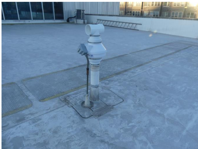
View of newly installed rooftop fan #F-3. This fan unit, Fantech model Rn4EC-4, is the recommended replacement for the older Fantech FR250 model.
