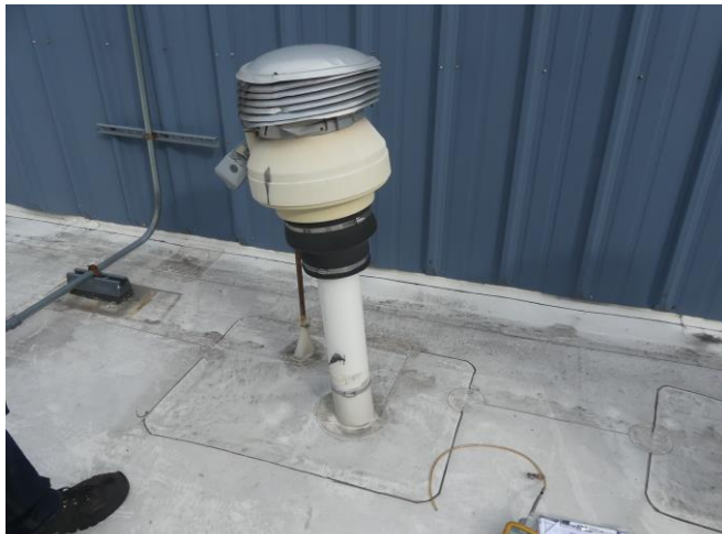
View of original rooftop fan #F-1, associated with the vapor extraction system (VES). This fan was observed to be damaged and operating poorly.
