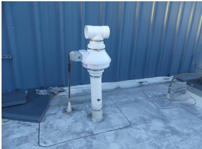
View of newly installed rooftop fan #F-1 (late October 2021). This fan unit, Fantech model Rn4EC-4, is the recommended replacement for the older Fantech FR250 model.
