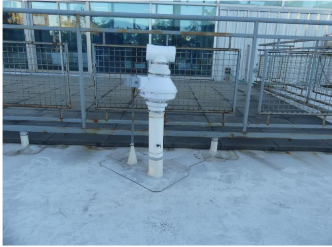
View of newly installed rooftop fan #F-4. This fan unit, Fantech model Rn4EC-4, is the recommended replacement for the older Fantech FR250 model.
