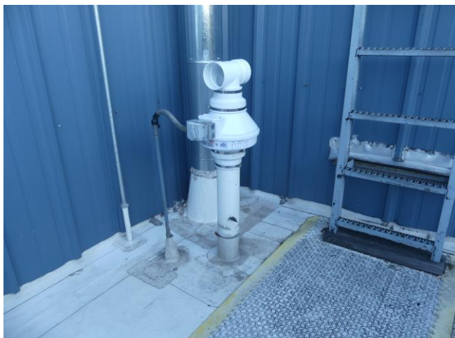
View of newly installed rooftop fan #F-2. This fan unit, Fantech model Rn4EC-4, is the recommended replacement for the older Fantech FR250 model.
