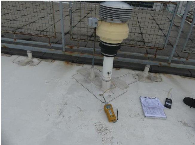
View of original rooftop fan # F-4, associated with the VES. This fan was observed to be operating properly.
