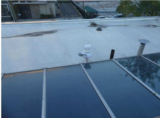
View of newly installed rooftop fan #F-5. This fan unit, Fantech model Rn4EC-4, is the recommended replacement for the older Fantech FR250 model.
