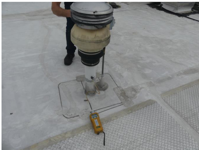
View of original rooftop fan # F-3, associated with the vapor extraction system (VES). This fan was observed to be damaged and operating poorly.
