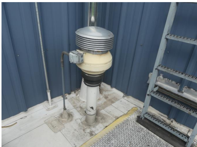
View of original rooftop fan # F-2, associated with the VES. This fan was observed to be operating properly.
