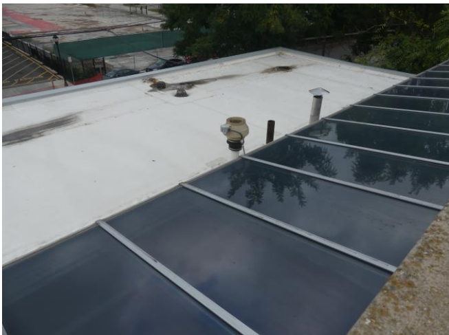
View of original rooftop fan # F-5, associated with the vapor extraction system (VES). This fan does not operate and serves as a passive extraction point.
