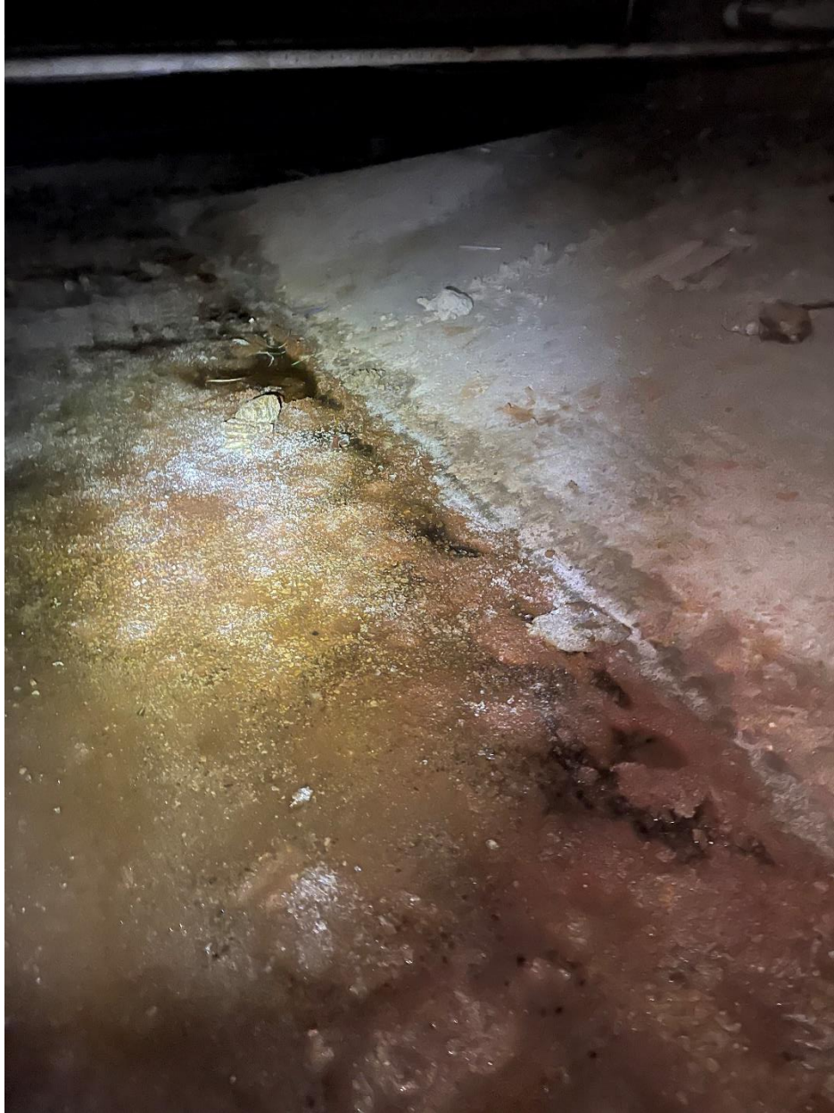
Photograph 8: Floor and sloped wall
