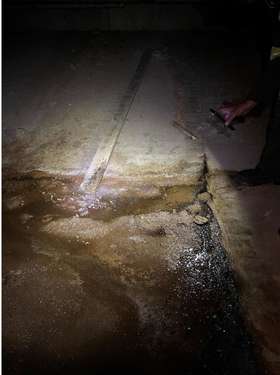
Photograph 10: Floor at corner of sloped wall.
