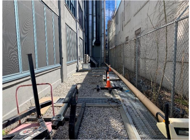
Former Drum Storage Area
