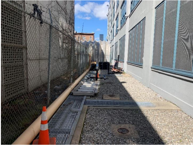
Former Drum Storage Area
