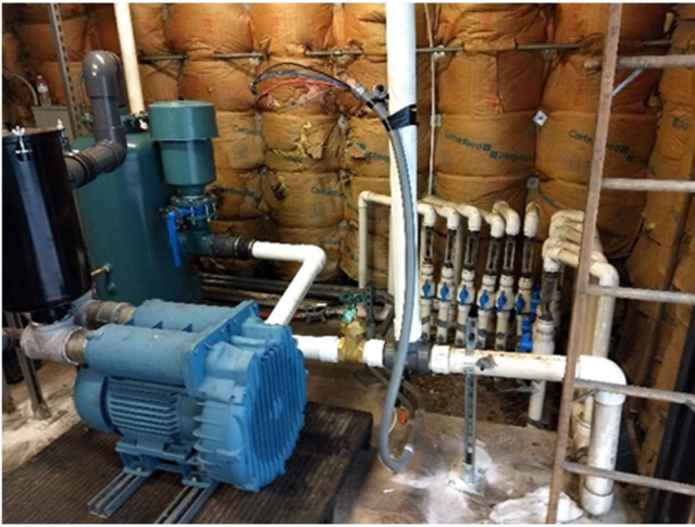
SSDS Blower and Legs in Treatment Shed
