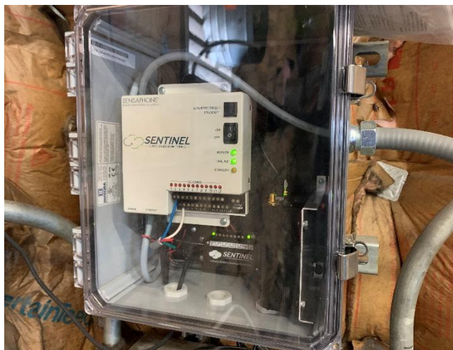
SSDS Telemetry and System alarm
