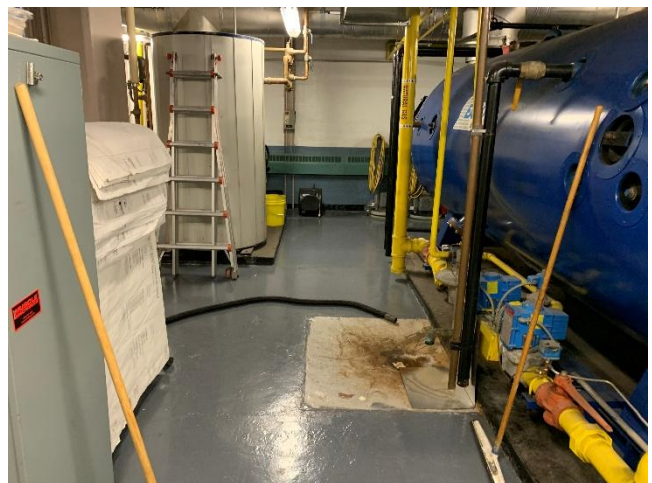
Basement Boiler Room
