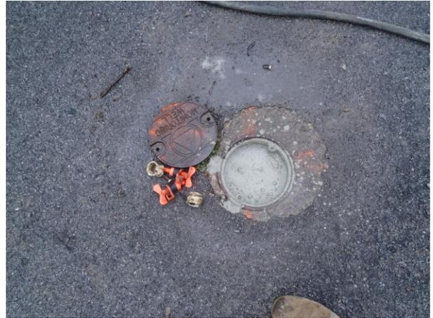
Photo 5: Well decommissioning – grout application (MW-6)
