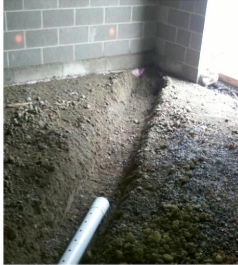
Photo 21: Sub slab depressurization system – Drain pipe layout
