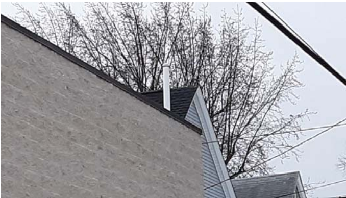
Photo 5: SVI Roof Vent – Northwest exterior building corner
