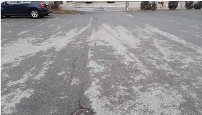
Photo 3: Main parking lot (looking northwest)
