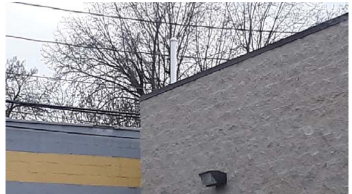
Photo 4: SVI Roof Vent – Southwest exterior building corner
