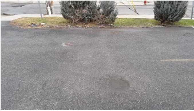
Photo 1: Parking Lot – Looking towards Kingston Place
