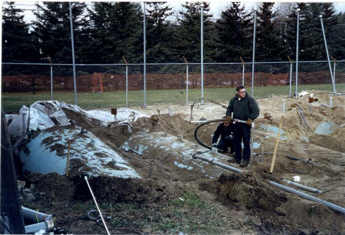
PHOTOGRAPH #6: USE OF DROP TUBE FOR REMOVAL OF RESIDUALS
