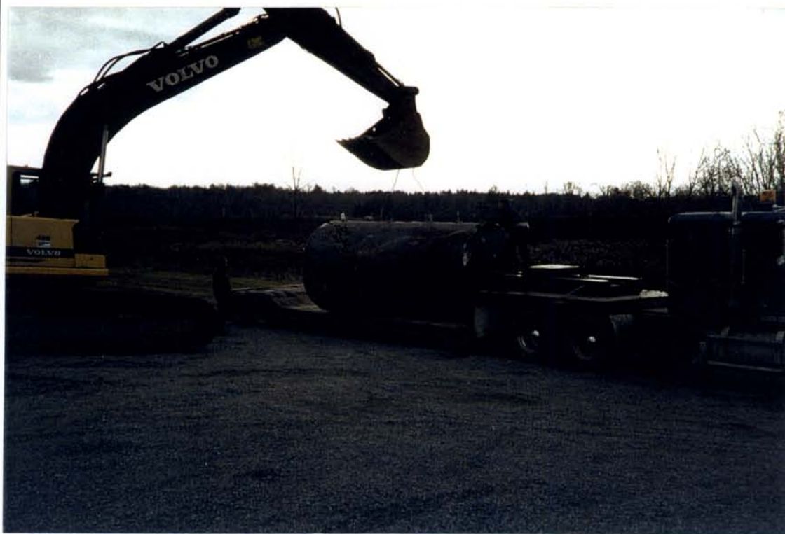
PHOTOGRAPH #10: TANK LOADING
