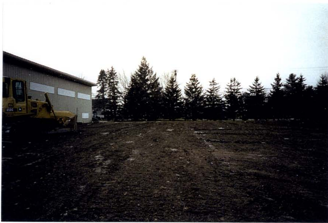
PHOTOGRAPH #15: SITE GRADING
