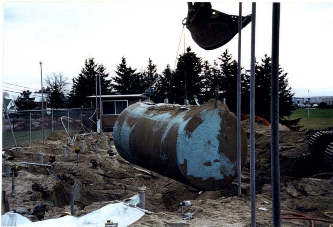
PHOTOGRAPH #9: TANK REMOVAL
