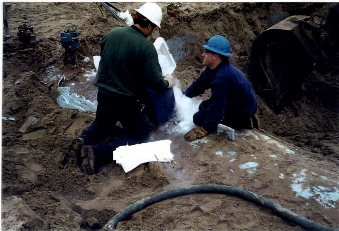
PHOTOGRAPH #7: DRY ICE APPLICATION
