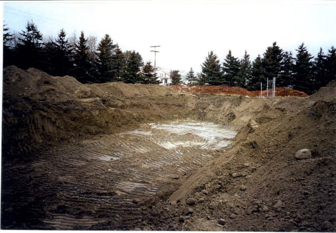
PHOTOGRAPH #13: COMPLETED EXCAVATION AND EXPOSED CONCRETE PAD
