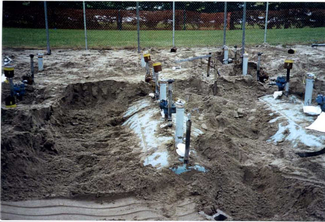
PHOTOGRAPH #5: EXPOSED TANKS
