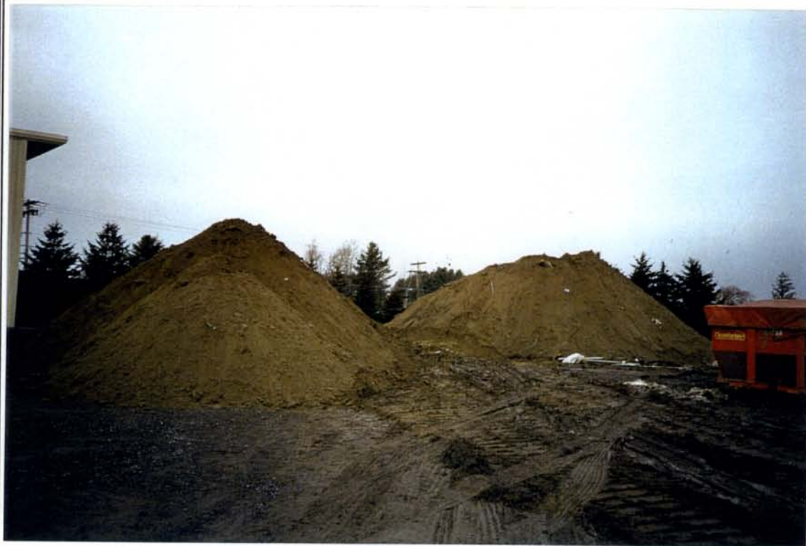
PHOTOGRAPH #12: STAGING OF NON-IMPACTED SOILS
