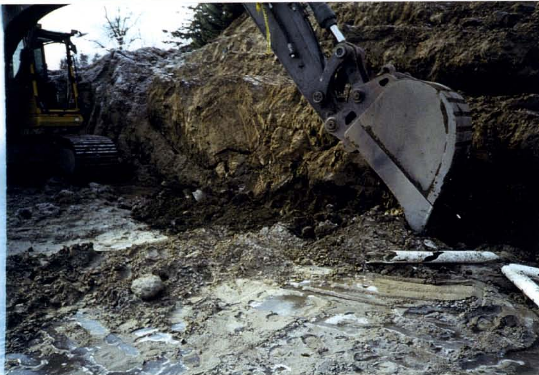
PHOTOGRAPH #14: EXCAVATION FOR CONFIRMATORY SAMPLING AROUND EDGE OF CONCRETE SLAB
