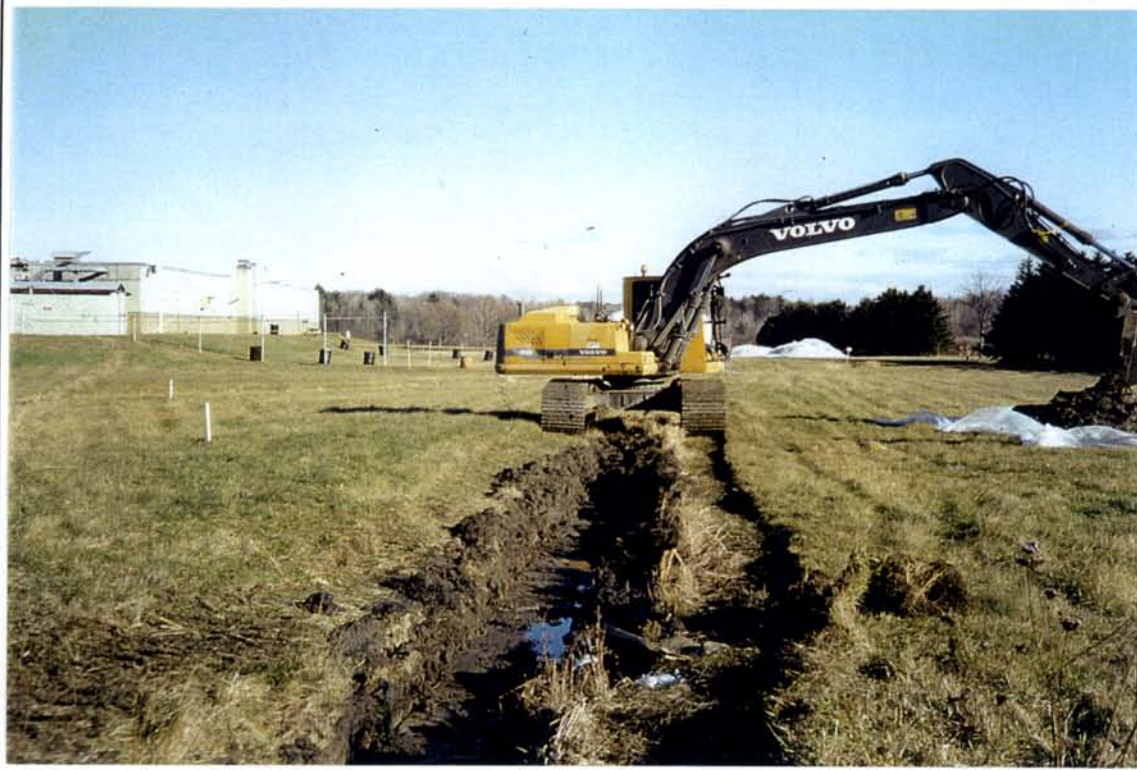
PHOTOGRAPH #17: EXCAVATION OF DRAINAGE SWALE
