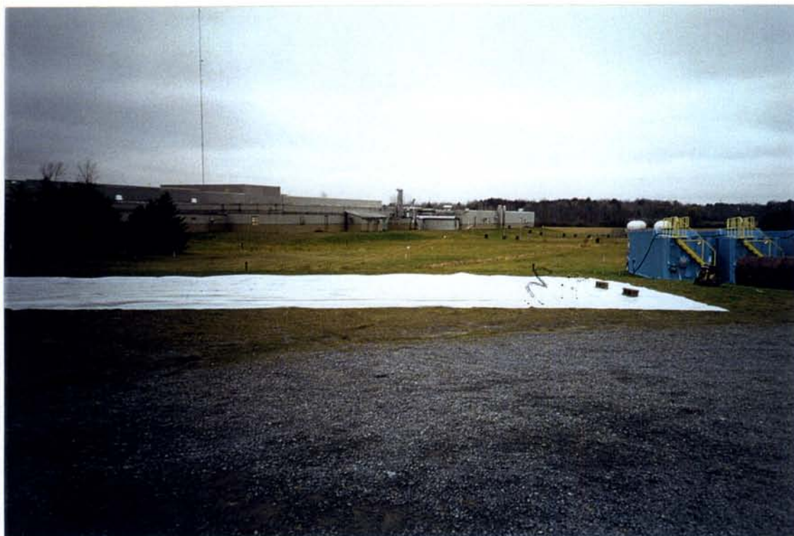
PHOTOGRAPH #4: POLYETHYLENE LINER
