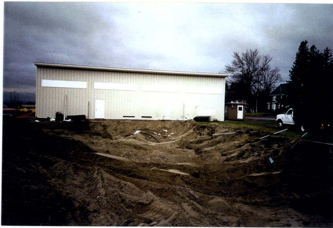
PHOTOGRAPH #11: EXCAVATION OF SOIL AFTER TANK REMOVAL
