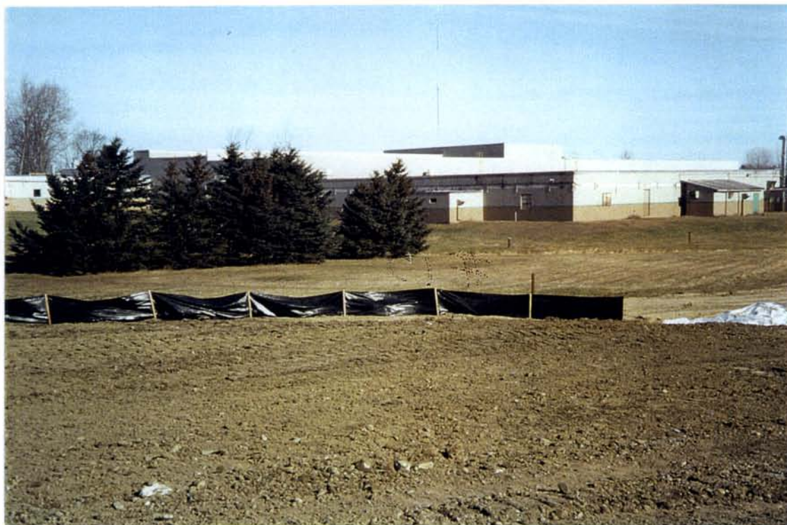
PHOTOGRAPH #16: SILT FENCING
