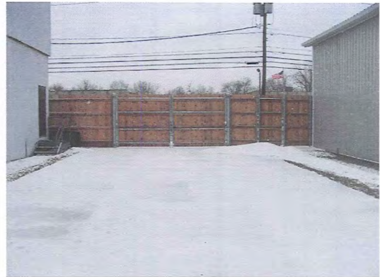
2. New cement pad facing west and Fillmore Ave
