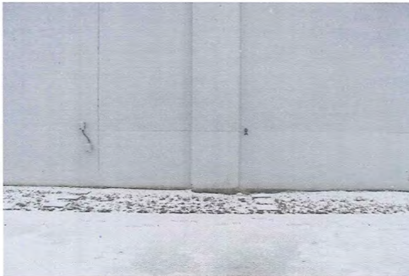
3. Location of where new sewer and water enters building
