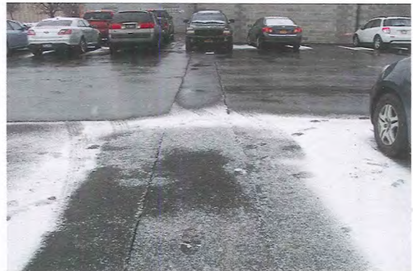
12 View of location of new water line towards parking lot and street utility connect
