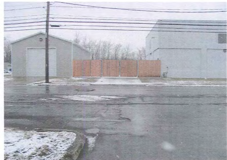
4. Location of new cement pad from Fillmore Street
