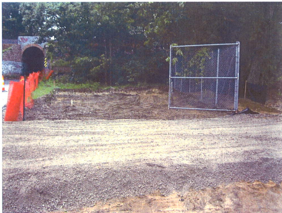
Construction entrance at River Road, showing partial 1-foot excavation area.
