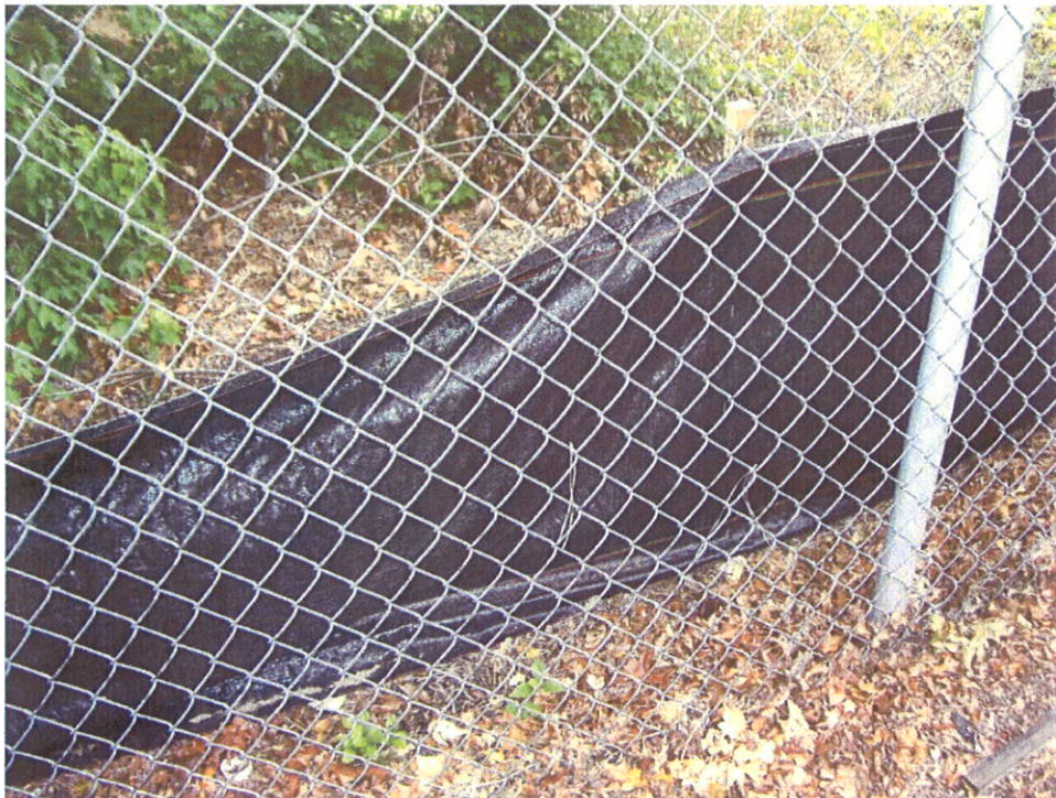
Completed silt fence, located along the fence line at the southwest of the fill area.
