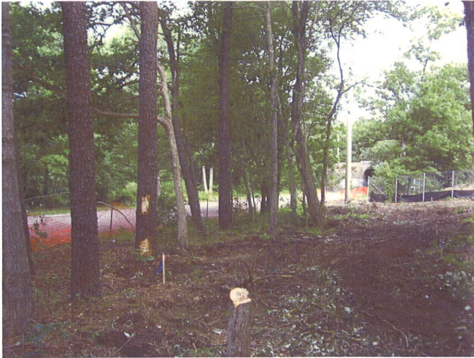
Drainage swale area post clearing and grubbing activities.
