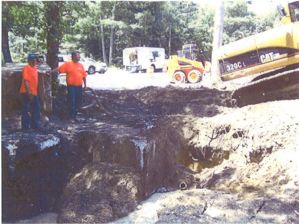
Excavation of the 6-foot area in the drainage swale, showing large concrete blocks.
