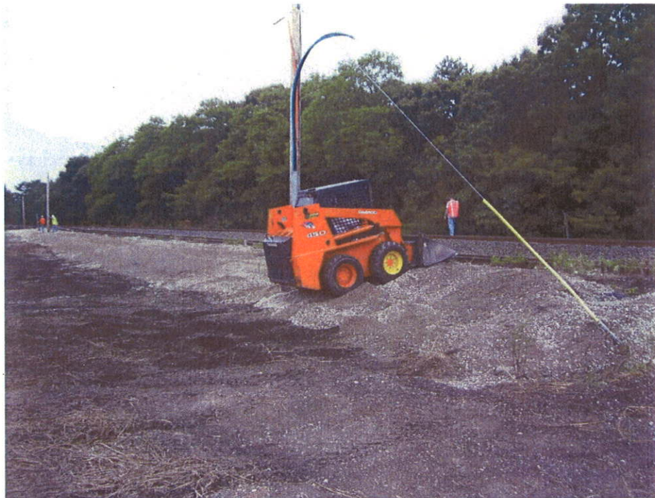
Fill area, showing the installation of the geotextile material and RCA.
