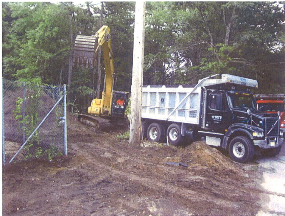
Live loading of contaminated soil in drainage swale area.
