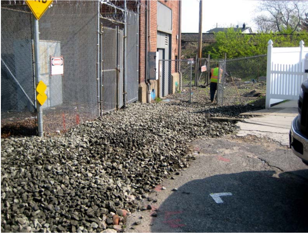
Stone installation area located south of the substation.
