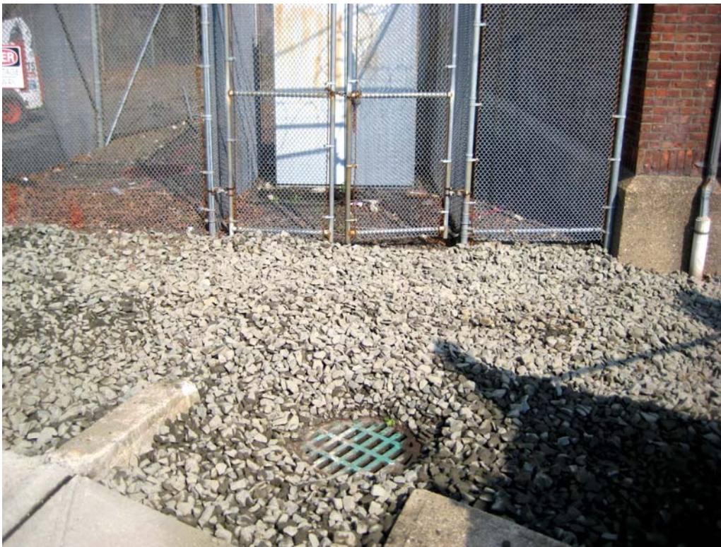
Stone installed in the non-fenced area south of the substation building.
