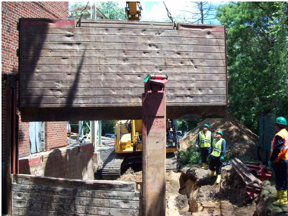
Installation of the sheeting at Area 2.
