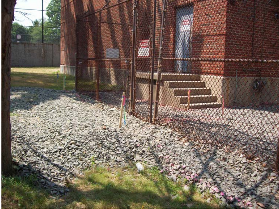
Southeast corner of the substation building, prior to remediation.
