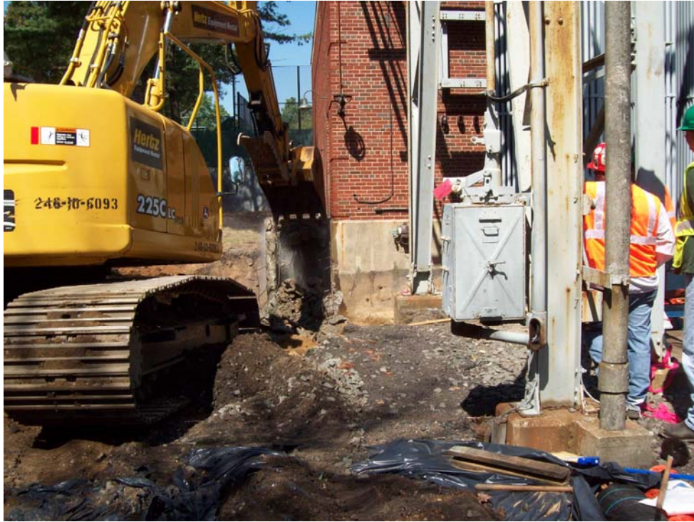
Demolition of the concrete platform and steps on the southeast corner of the substation building.
