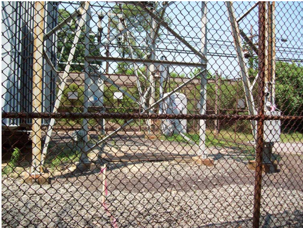
Transformer yard area, prior to remediation.
