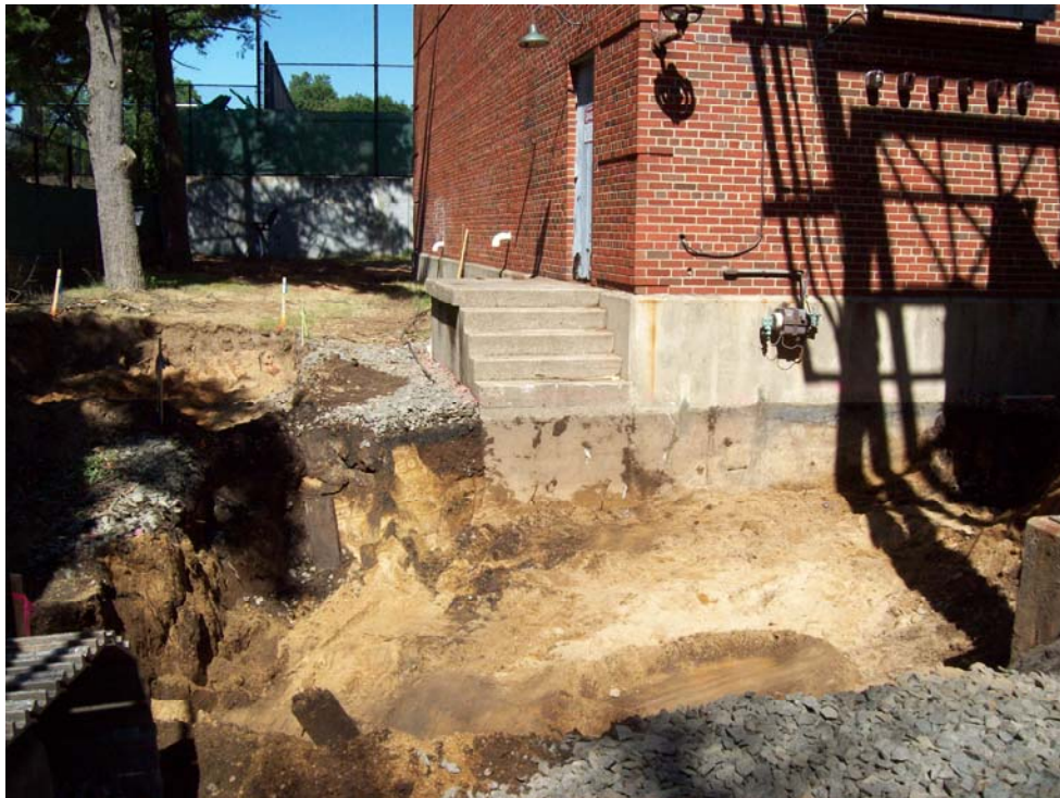
Completed Areas 1 and 3, prior to the excavation of Area 2.
