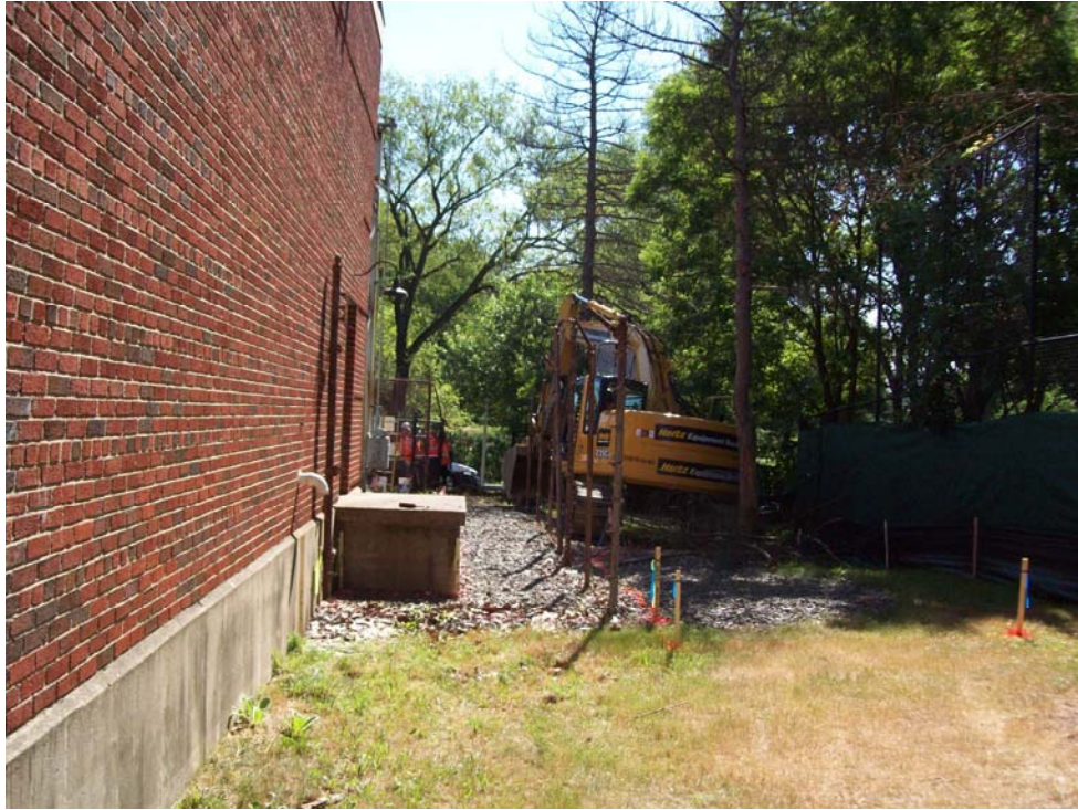
Southeast corner, during transformer yard fence removal.
