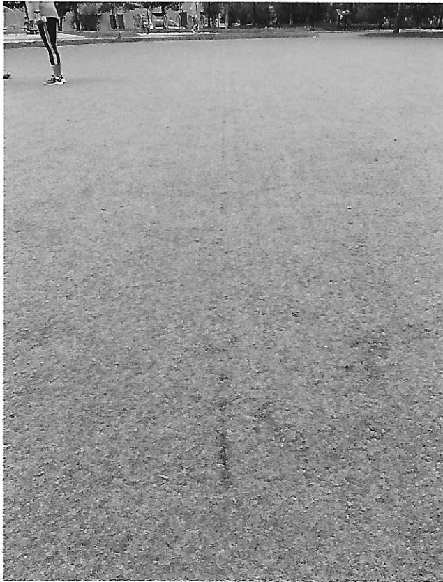
Photo 5 – Tear in Artificial Turf
