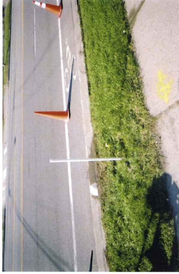
Off-site groundwater sampling - BH-01. Typical temporary piezometer installation.
