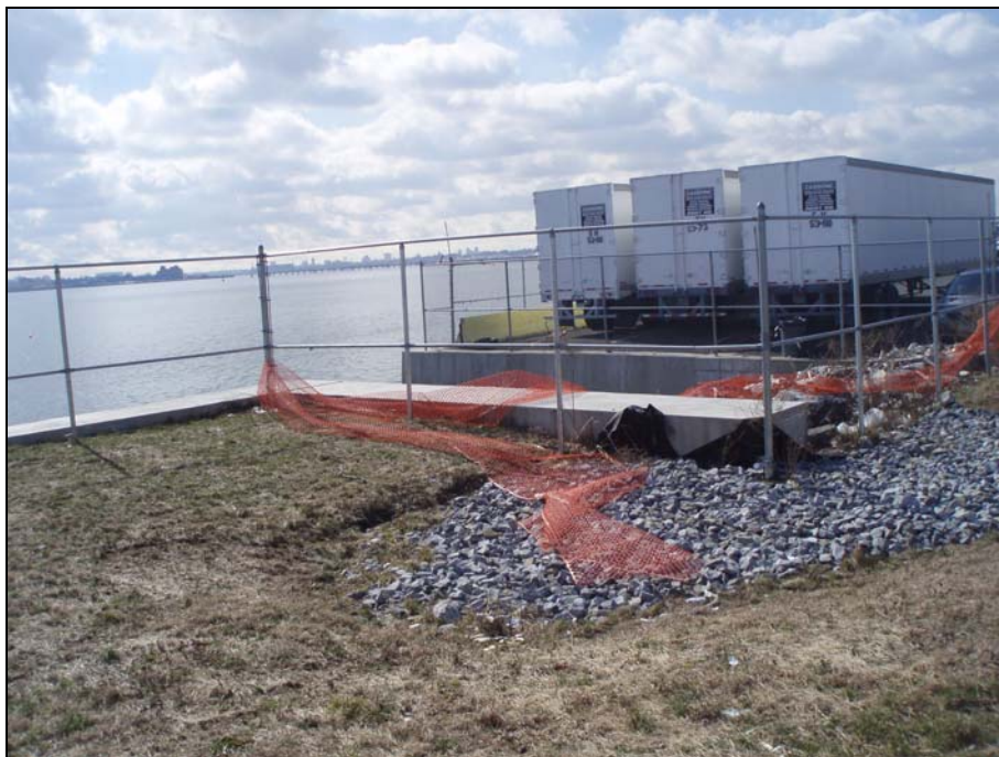
Photograph No. 23 – Portion of Perimeter Site extending into Site C OU-2, Rip-rap upon pipe entering river (looking south)
