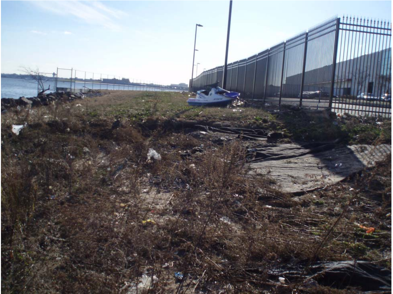
Photograph 1: Erosion noted in the partially constructed greenway section; located at the northwest corner of the site (looking south). Sea-Doo seen in the picture had no gas tank, motor or battery (no spill condition noted).
