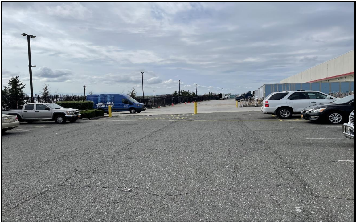
Photo 2: Facing southwest in the eastern portion of the Site; engineering controls (asphalt pavement and concrete slab) are still in place and in good condition in the truck loading area.
