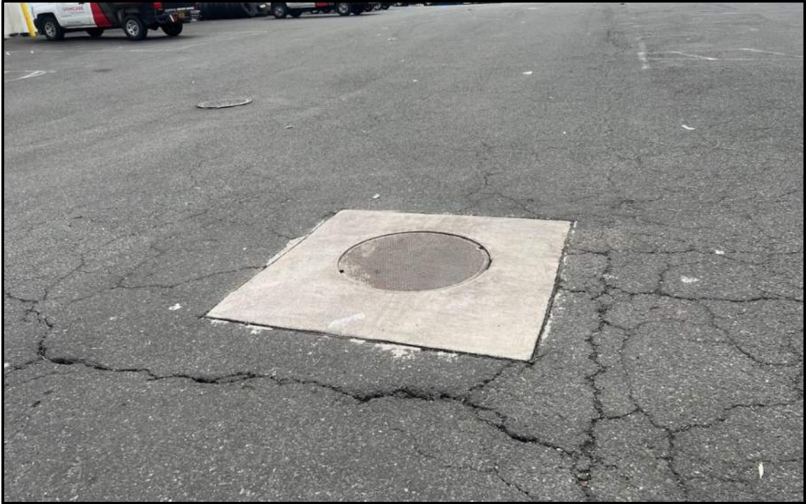
Photo 5: Facing east along the southern portion of the building; area where manhole was reset and repaved. Minor cracking in the asphalt around the manhole.
