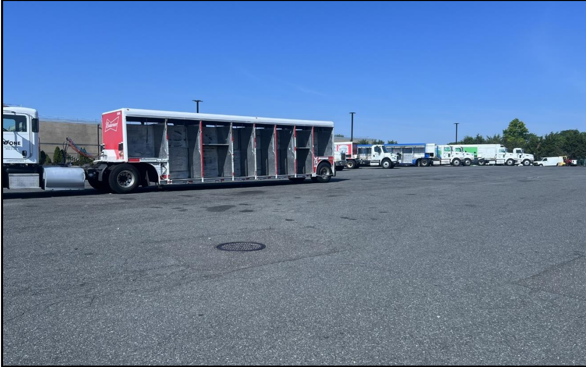
Photo 5: Facing southwest in the southern paved parking area of Parcel C; asphalt in fair condition with evidence of minor cracking, as well as former utility and pavement repairs.
