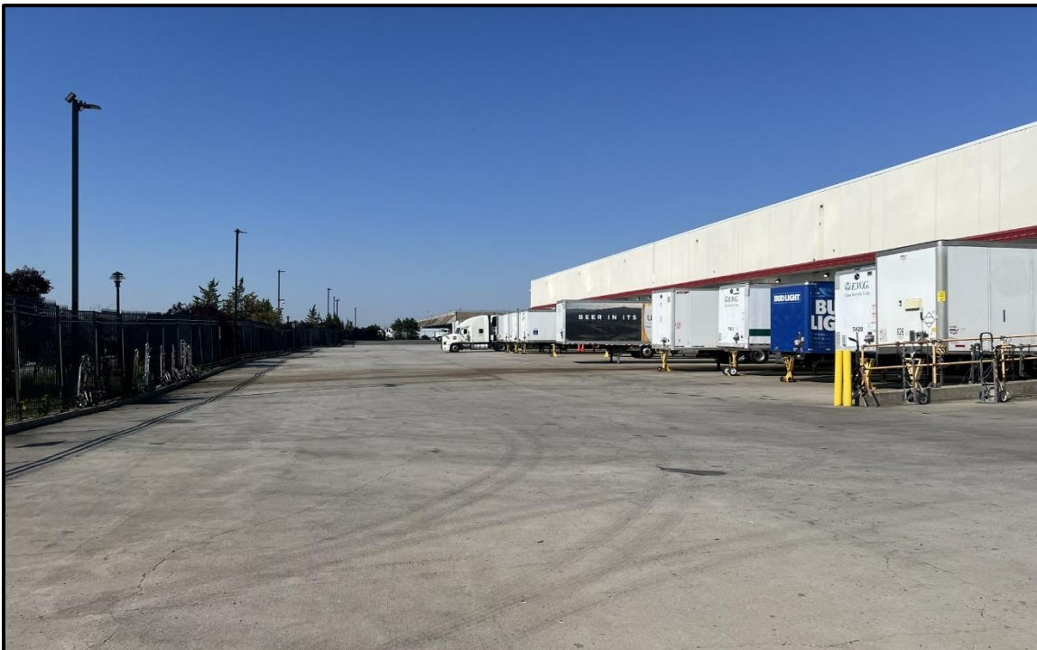
Photo 2: Facing southwest in the eastern truck loading area of the Site; reinforced concrete slab in fair condition with minor asphalt cracking noted.
