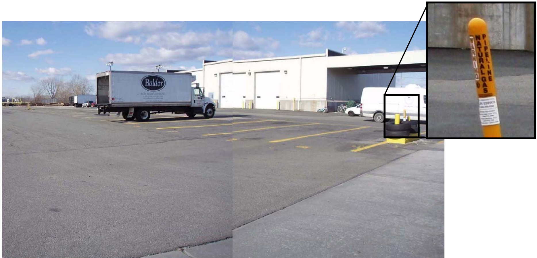
Photograph No. 7 – Site E OU-1: Marker for Consolidated Edison of New York easement and 24-inch gas line and saw-cut asphalt associated with gas line-installation and maintenance (looking north-northwest)
