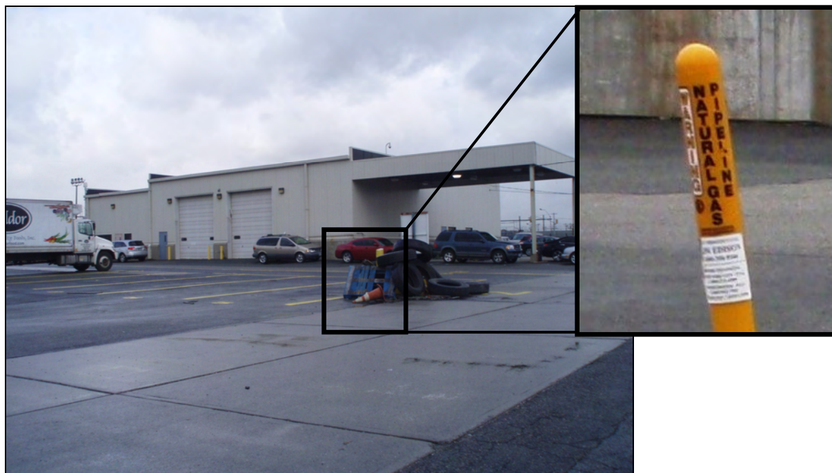
Photograph No. 7 – Site E OU-1: Marker for Consolidated Edison of New York easement and 24-inch gas line and saw-cut asphalt associated with gas line-installation and maintenance (looking north-northwest)
