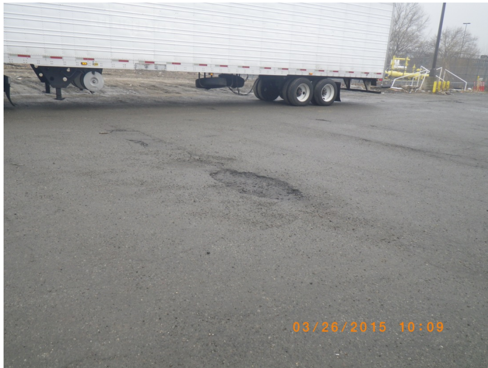
Photograph 7 – Site E-OU1 Example of pot hole that will be repaired (looking northwest)
