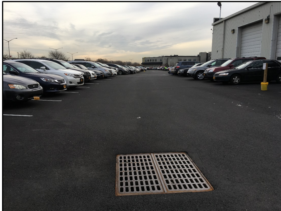
Photo 8: Facing east in the northern portion of the site; area around the storm drain repaired via re-paving of the parking lot (January 2020 inspection).
