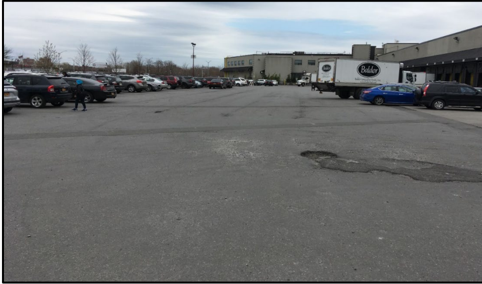
Photo 9: Facing east in the northern portion of the site; pothole observed in one of the heavily trafficked areas of the Site.
