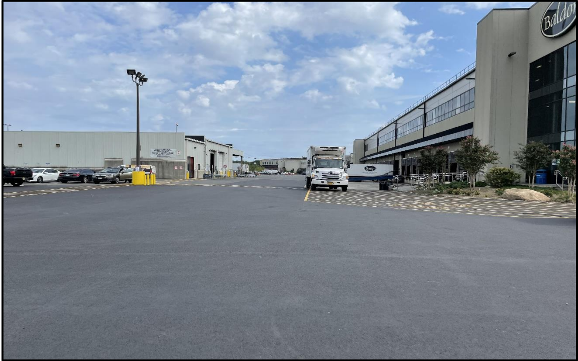
Photo 1: Facing east in the northern portion of the site; engineering controls (asphalt and building) are in place and in good condition.
