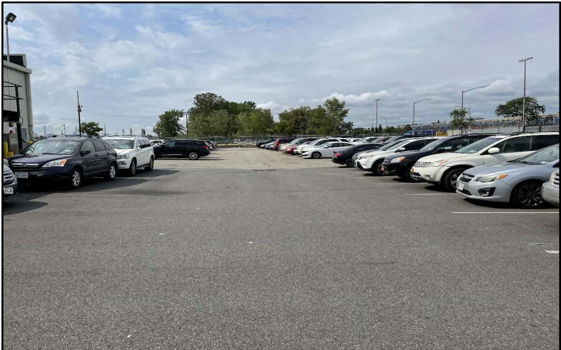
Photo 4: Facing west in the northern portion of the Site; engineering controls are in place and in good condition within the employee parking area.
