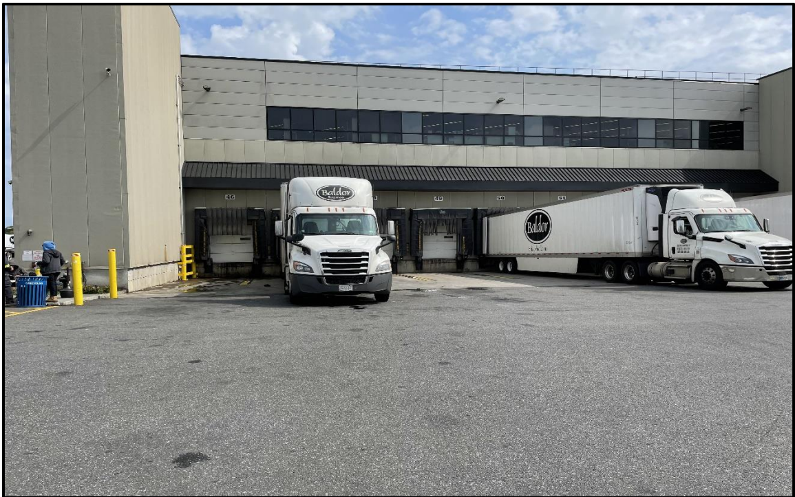
Photo 2: Facing east in the western portion of Site E OU-1; asphalt and reinforced concrete slab in the western truck loading dock in good condition.
